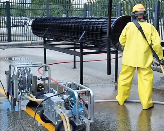
Semi-automated water jet systems have been helping chemical plants and refineries improve productivity for many years. For example, high-pressure water jetting is a very effective way to blast hard deposits out of heat exchanger tube bundles, and to remove build-up from a bundle's exterior, or shellside. Years ago, an operator would manually feed a flexible lance into each tube in turn, and activate the water flow with a foot control.
