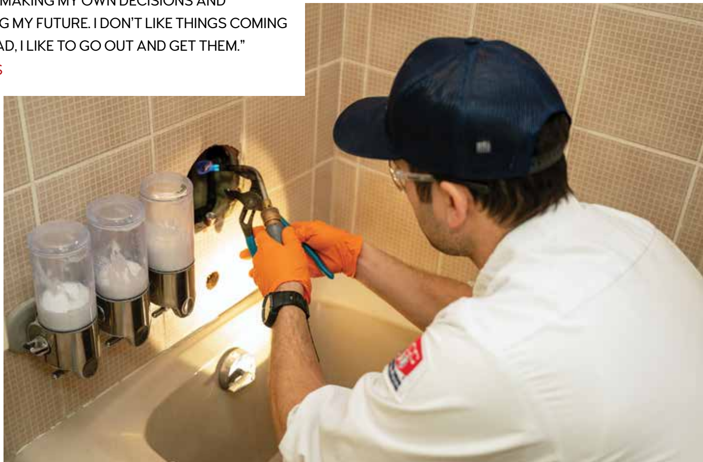
» Kyle Stong solders pipe while on a bathroom project.
