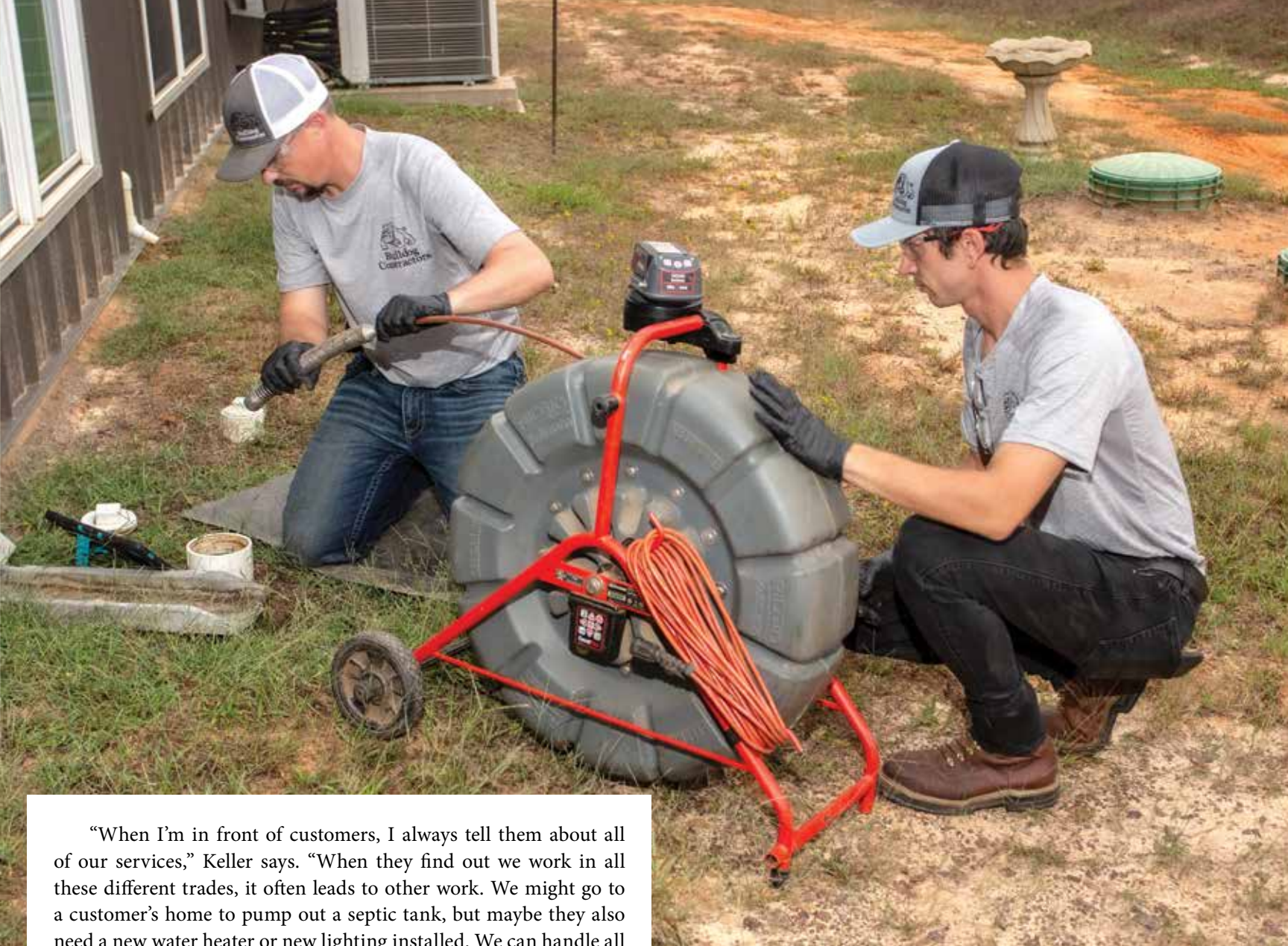
▲ Jeff Keller and Nathan Harrah inspect a drainline through a clean-out using a RIDGID SeeSnake pipeline inspection camera.
