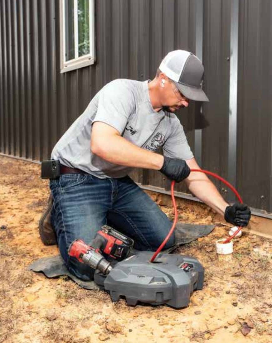
▲ Jeff Keller uses a RIDGID FlexShaft machine on a drainline.
