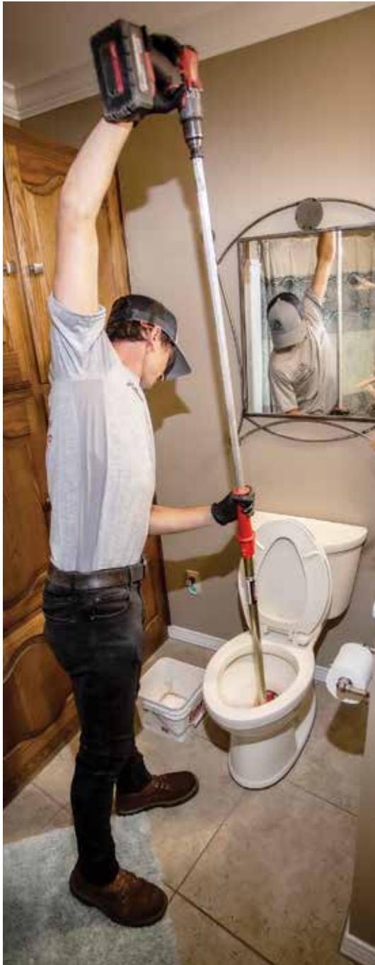
▲ Nathan Harrah uses a RIDGID toilet auger.
