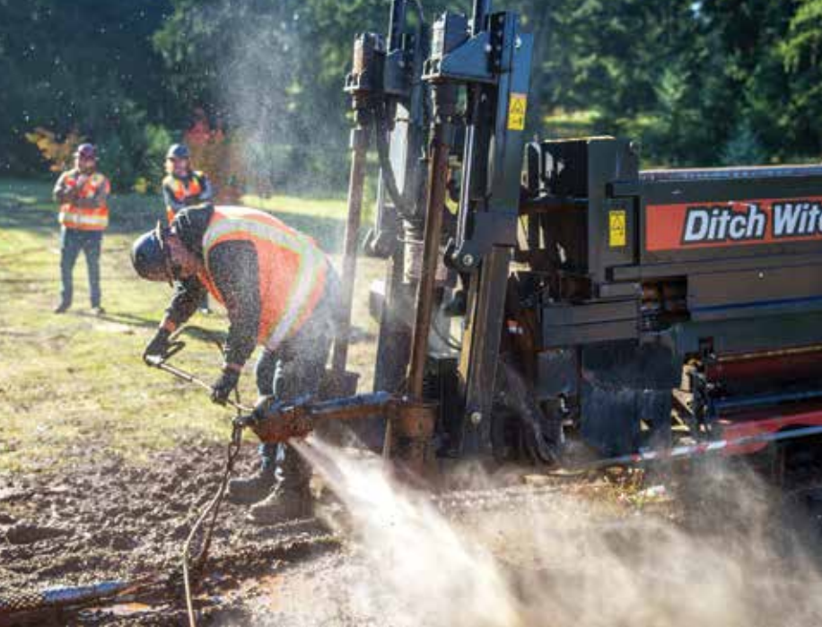
Stephen Dahlstrom cleans the drill head of a Ditch Witch JT20.
