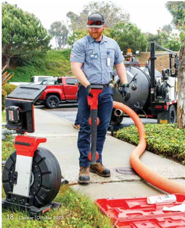
✓ Nicholas Garside, technician manager for Hansen's Plumbing, uses a Milwaukee Tool M18 120-foot Mid-Stiff Pipeline Inspection System and M18 Locator to verify a clean-out prior to repairs at a commercial property in Carpinteria, California.
