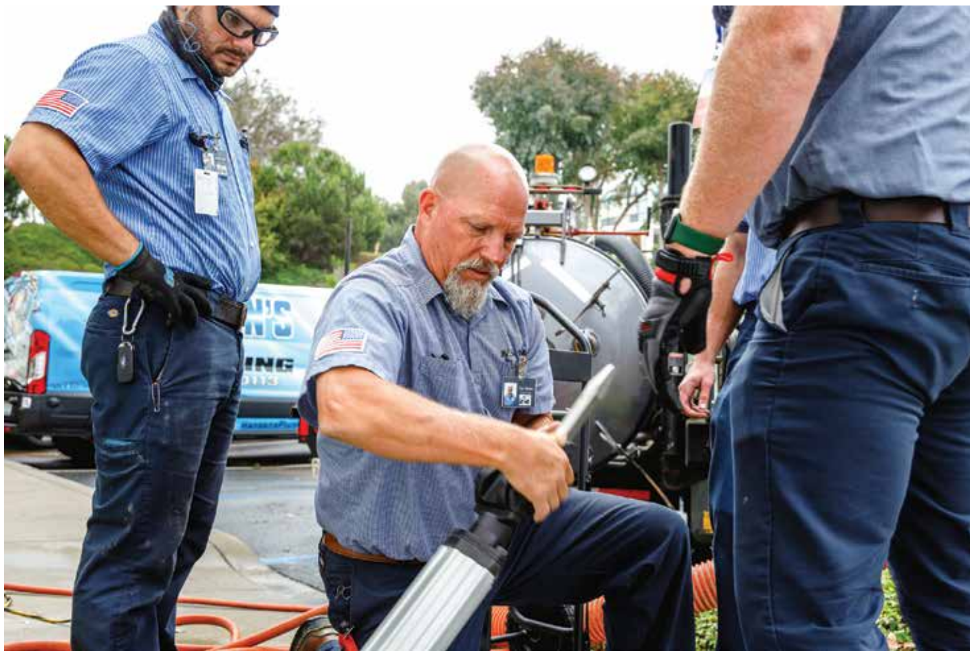
✓ Nicholas Garside, technician manager for Hansen's Plumbing, uses a Milwaukee Tool M18 120-foot Mid-Stiff Pipeline Inspection System and M18 Locator to verify a clean-out prior to repairs at a commercial property in Carpinteria, California.
