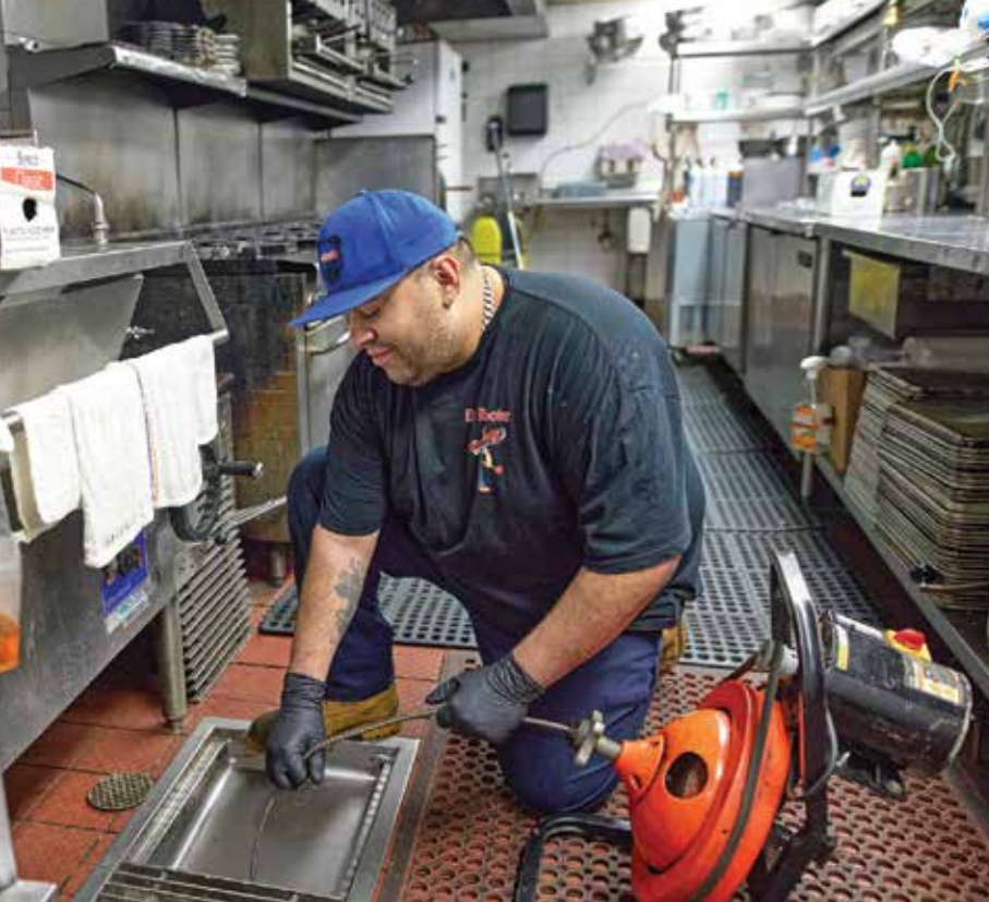
Technician George Vargas uses a Mini-Rooter XP from General Pipe Cleaners, the machine the company breaks out to tackle the smallest lines.
