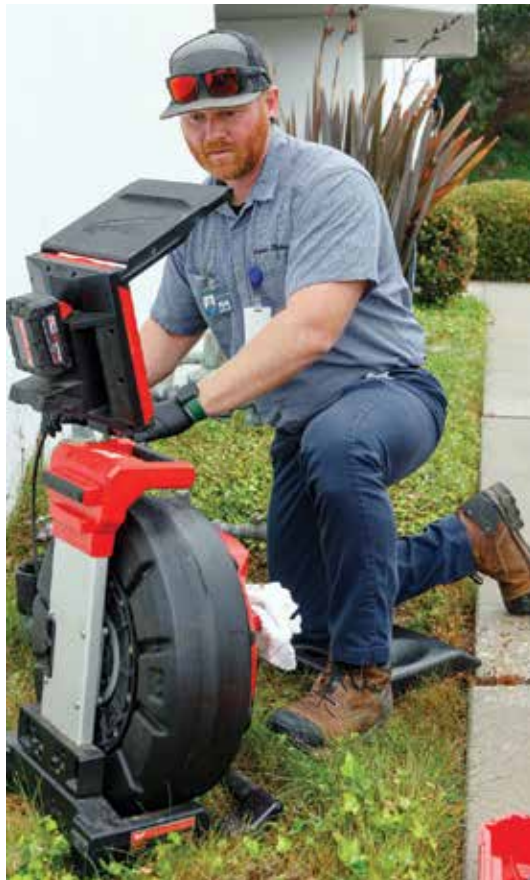
Garstide verifies a cleanout with a Milwaukee Tool M18 120-foot Mid-Stiff Pipeline Inspection System.
