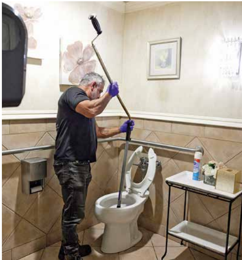
◀ Tony Garcia works on a clog through a toilet access.
