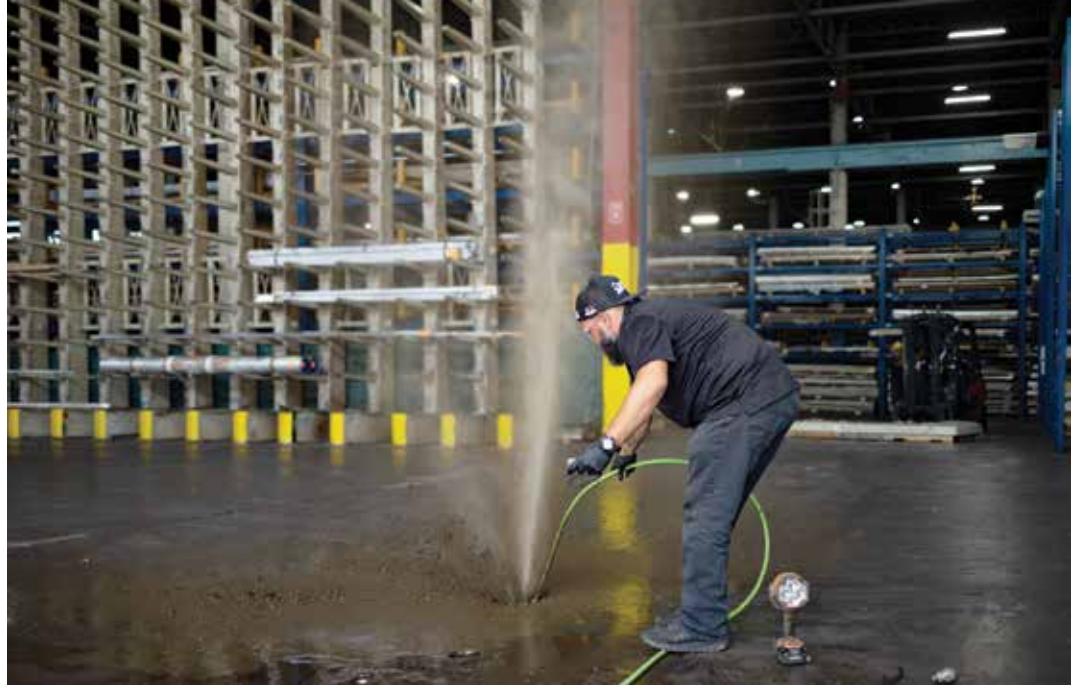
➤ Juan Roman jets a line. Daniels Plumbing likes to use Spartan 738 skid-mounted jetters.
