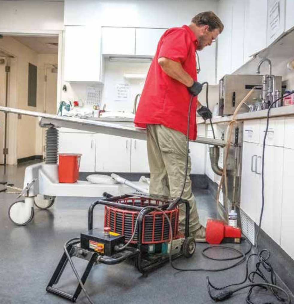
📍 Rodney King cleans a drainline for the embalming table at a funeral home.
