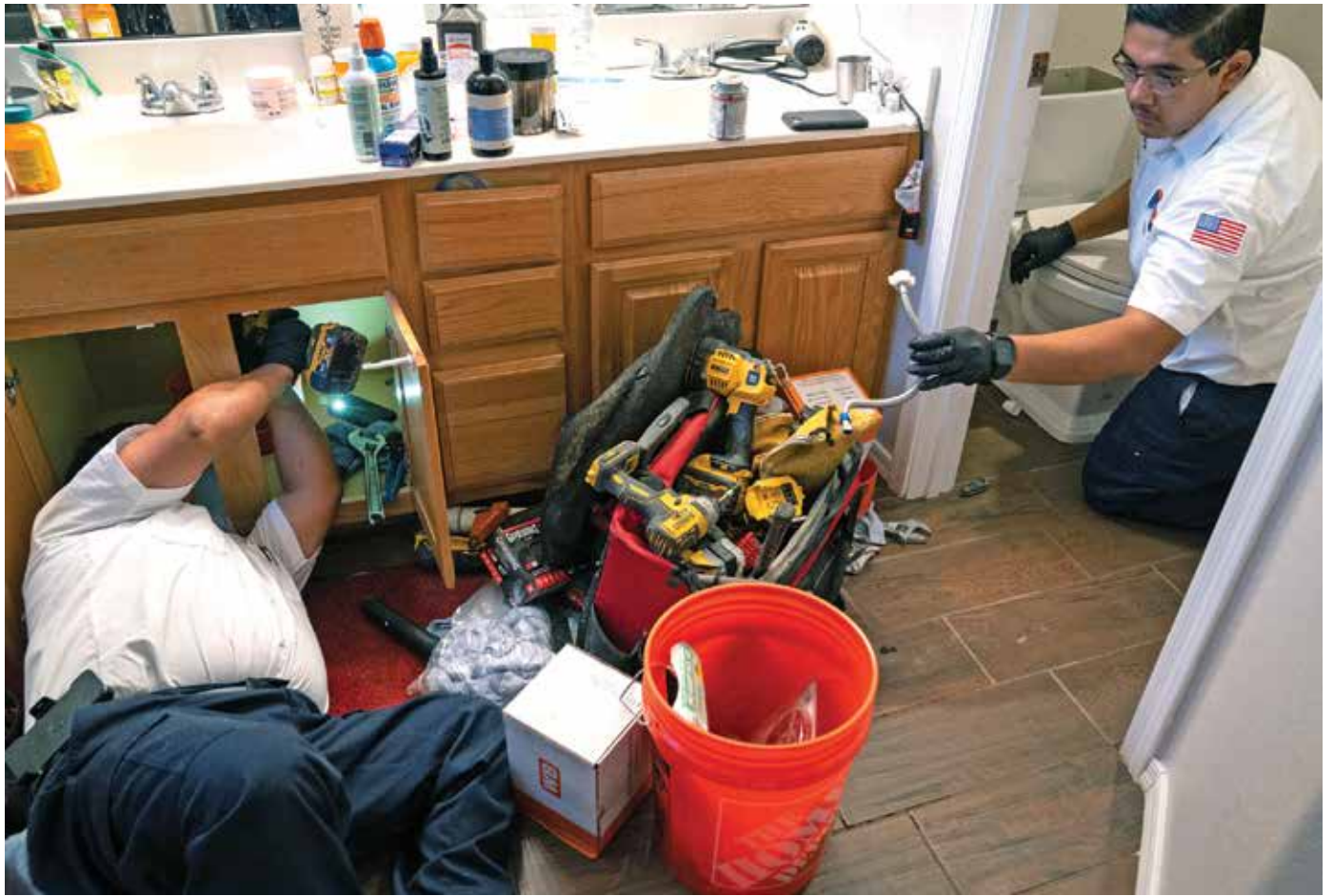
» Scottin McCabe and Bryan Estrada do work in a bathroom.
