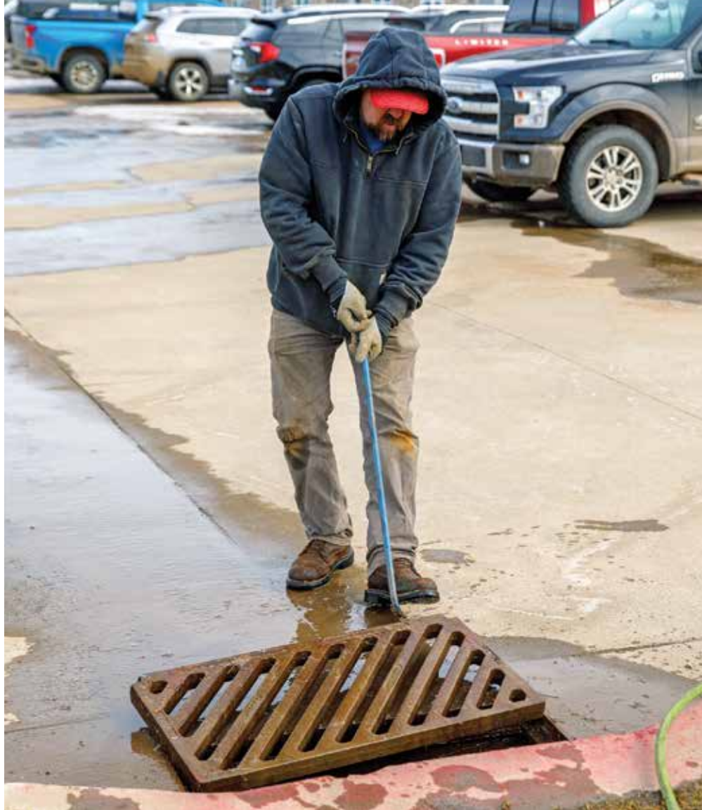
▲ Burris uses a sledgehammer and crowbar to loosen a storm drain prior to jetting it. The drain had become clogged with ice so Burris used boiler-heated water to clear the blockage.
