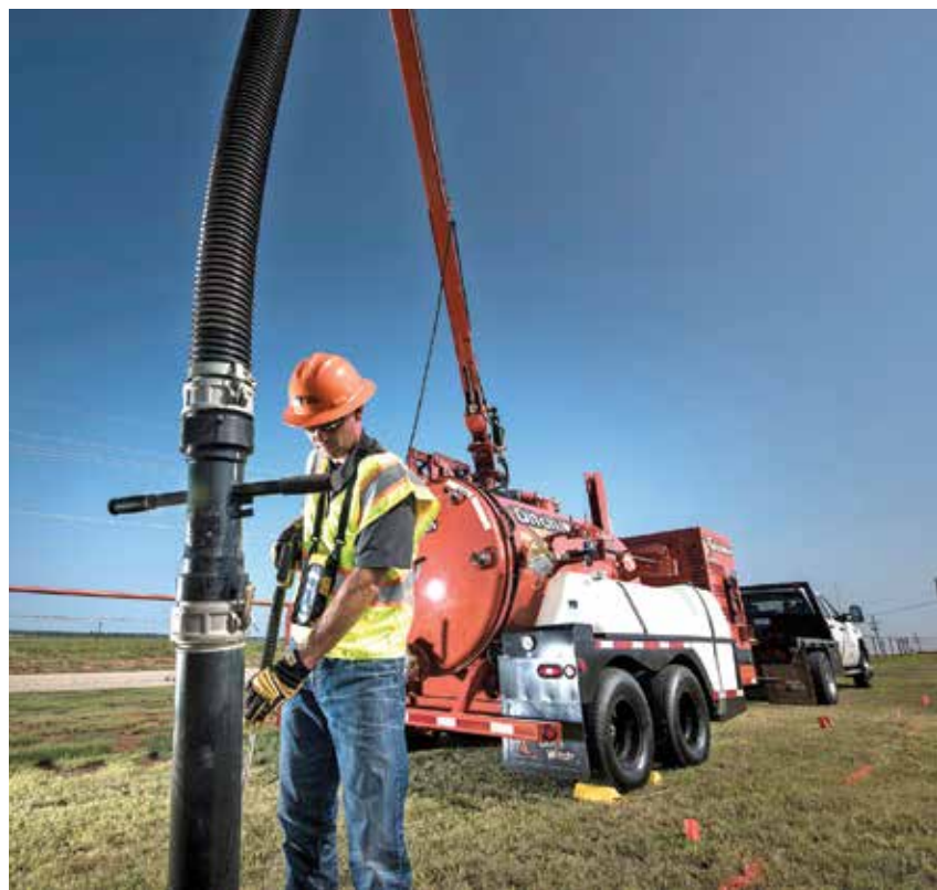
▲ Vacuum excavation has become a go-to method for many for locating and avoiding damage of underground utilities. (Photos courtesy of Ditch Witch)
