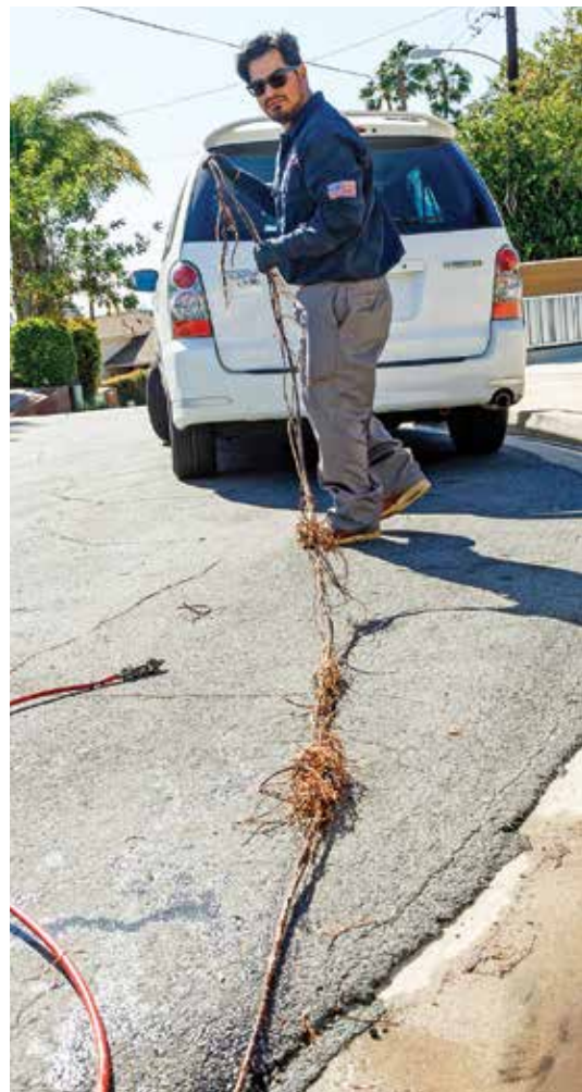
⚡ Rodriguez removes a long root ball severed with a RIDGID FlexShaft K9-204 snake on a residential job in San Diego.
