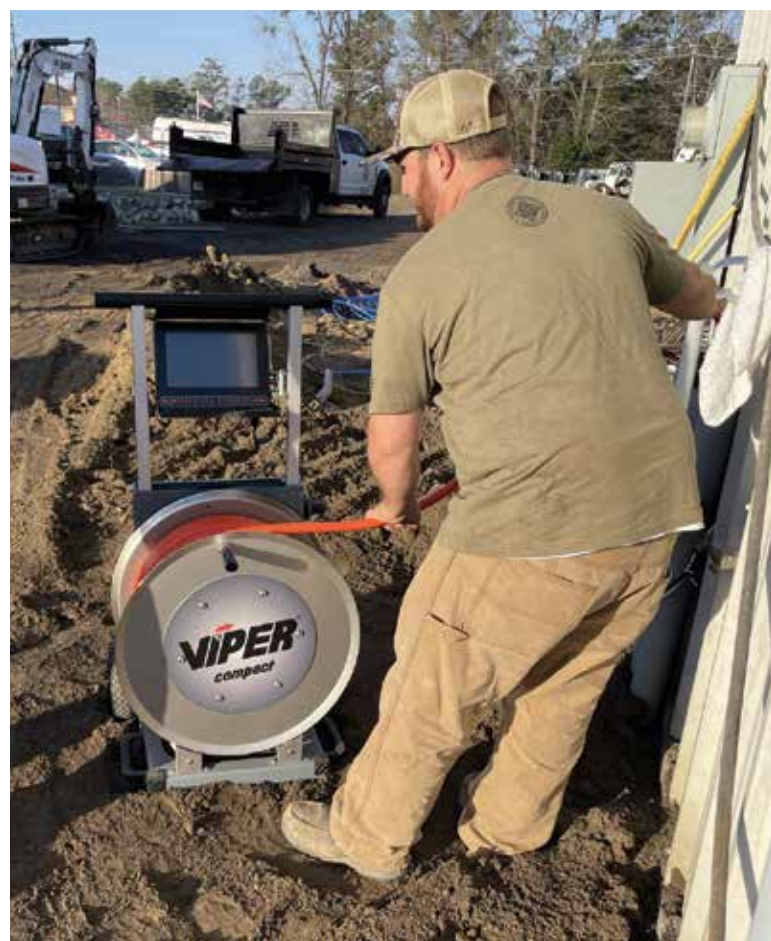
▲ Mason Powell, a technician for Stokes Plumbing & Trenchless, uses a Viper combination camera and jetter to inspect and clean a 36-inch-diameter stormwater sewer at a business in Georgia.
