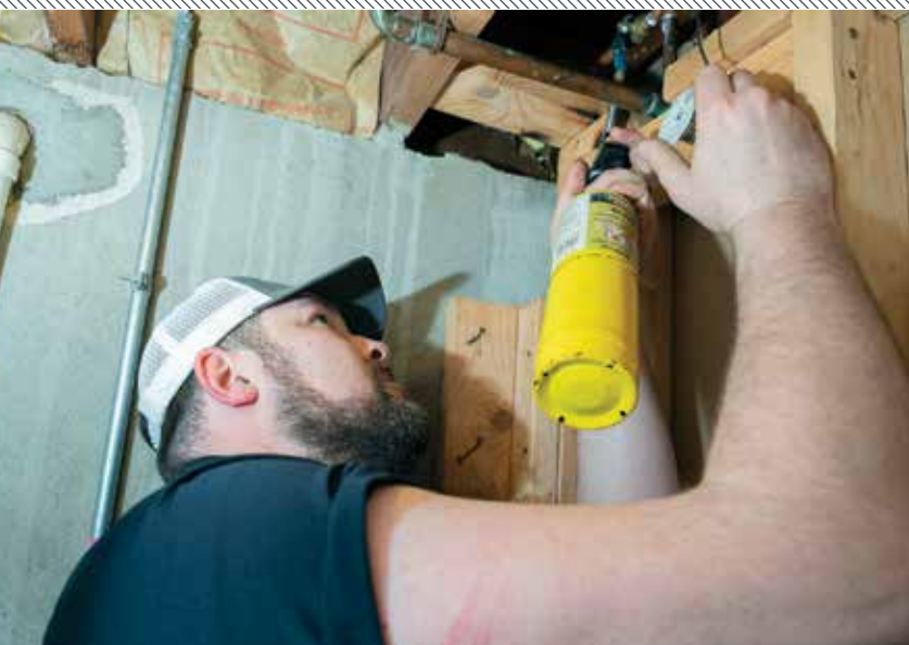
« Wilburn solders copper pipe while doing a hose bib replacement job.
