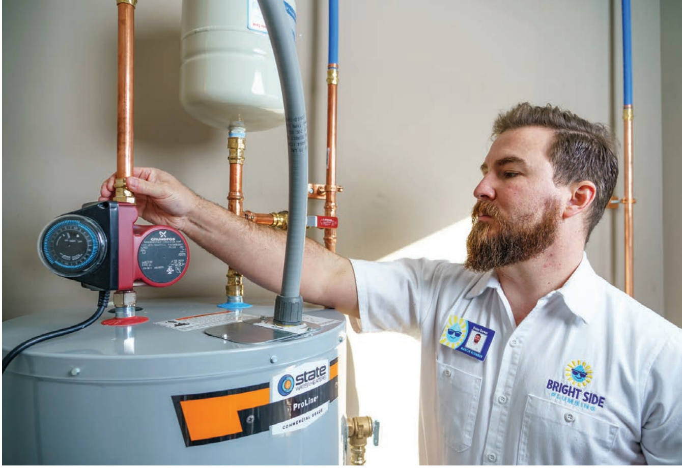
«Barker checks the compression fittings just above the circulation pump (Grundfos) during a water heater installation.
