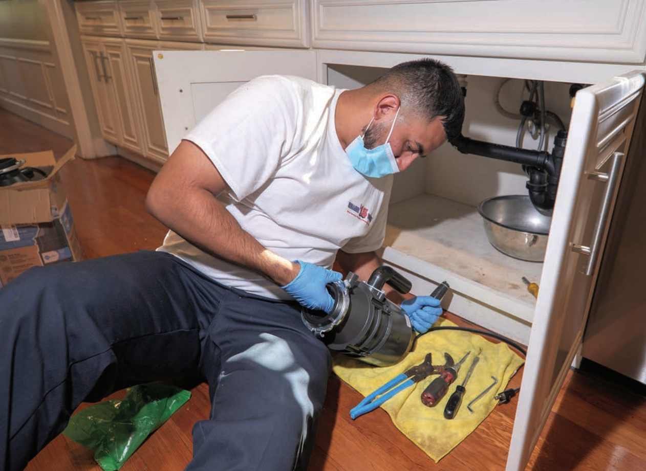
« Charlie Morales replaces a garbage disposal in a residence.
