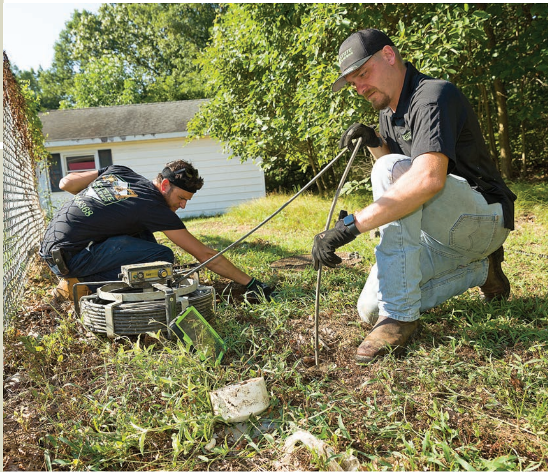
Mike Kraemer and Steve Russo use an EasyCAM E5200 camera to inspect a septic system at a home in New Egypt, New Jersey.
