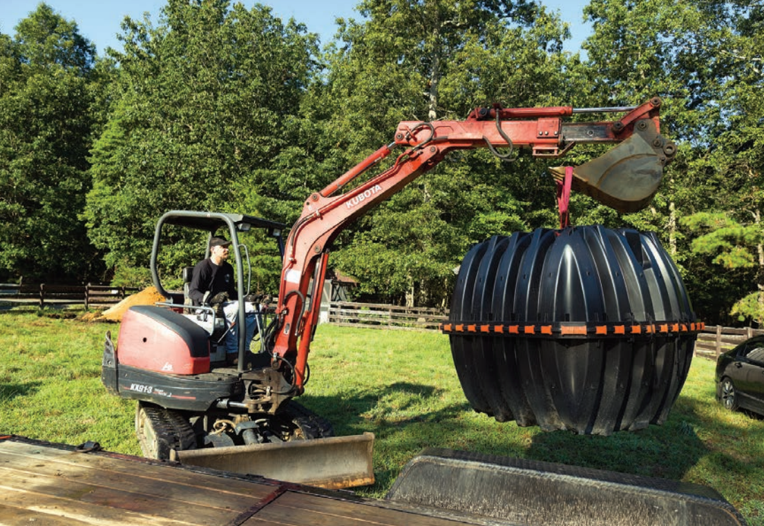
◀ Steve Russo prepares to install a new Infiltrator IM-540 septic tank on a job in New Egypt, New Jersey.
