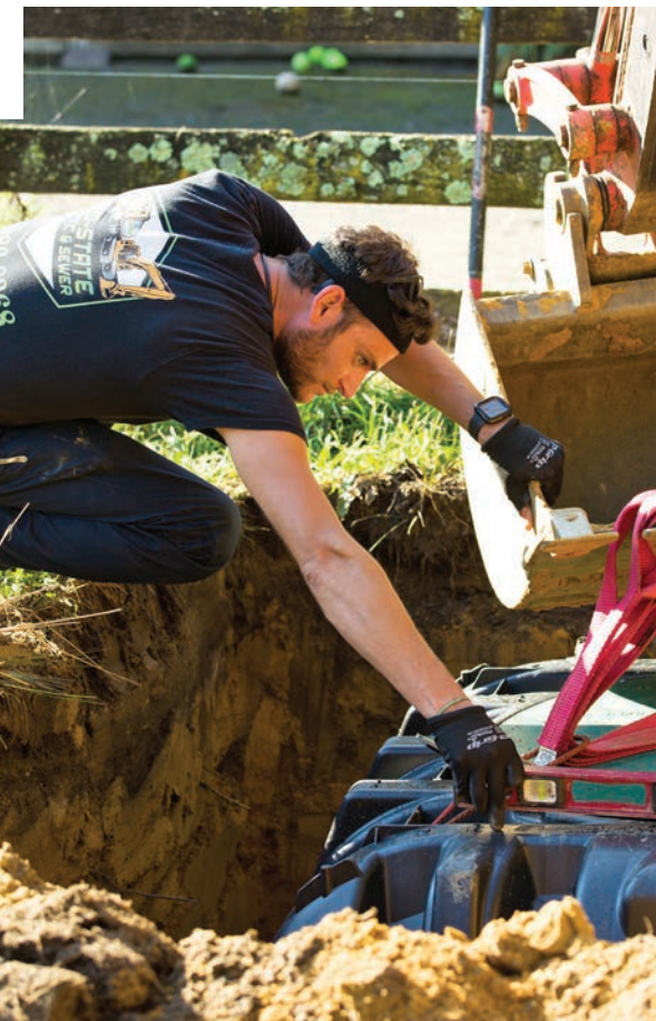
✔ Laborer Mike Kraemer levels the new Infiltrator IM-540 septic tank.
