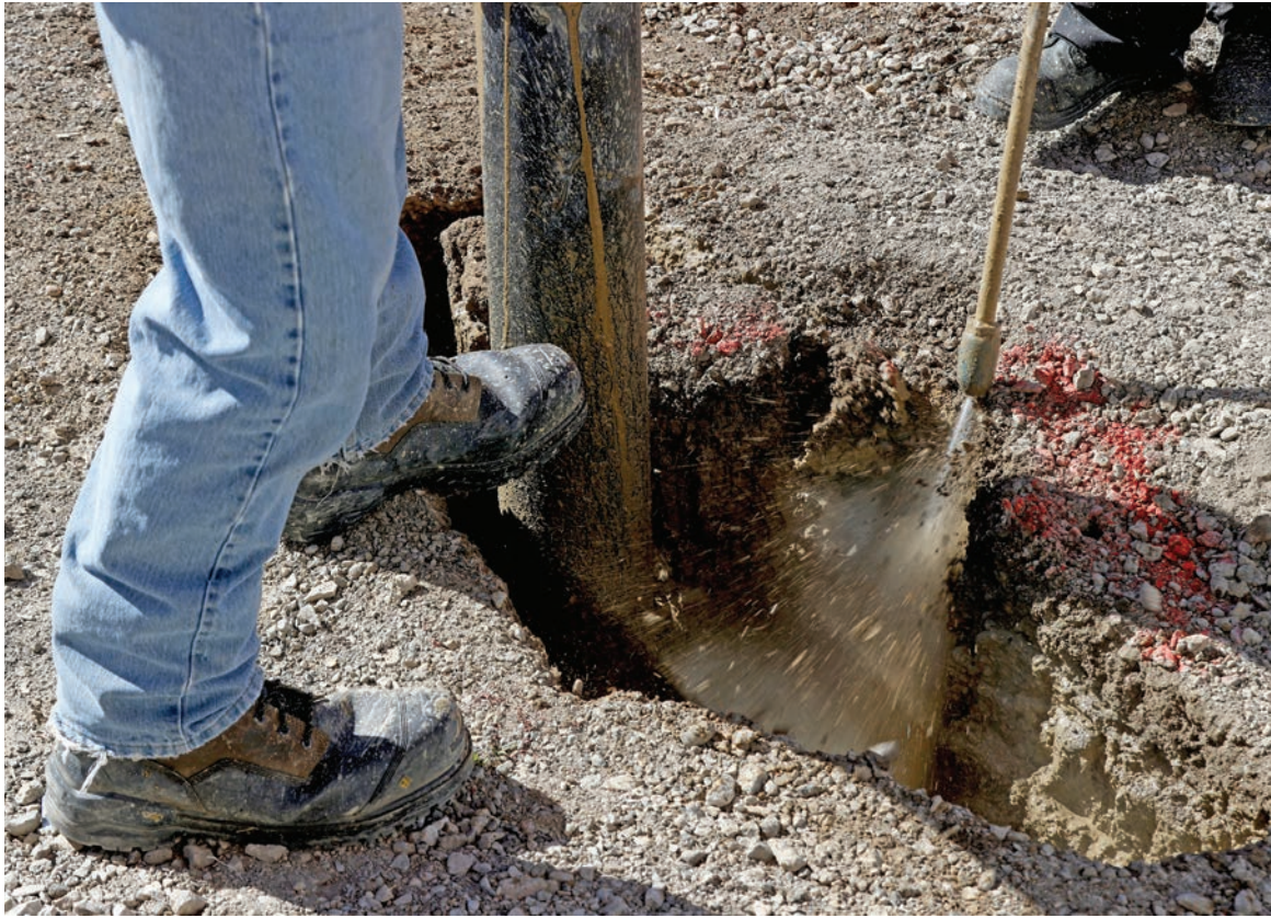
Technicians hydroexcavate to expose a utility line at a job site.
