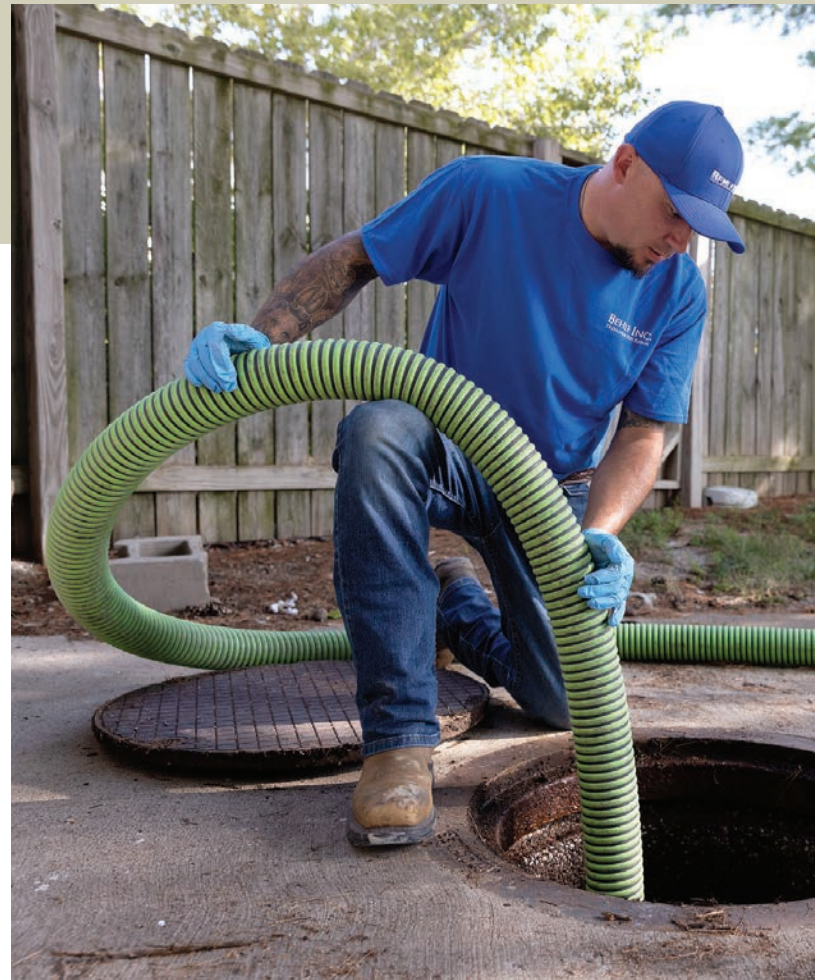
↘ McDowell pumps out a grease trap on a commercial job site.
