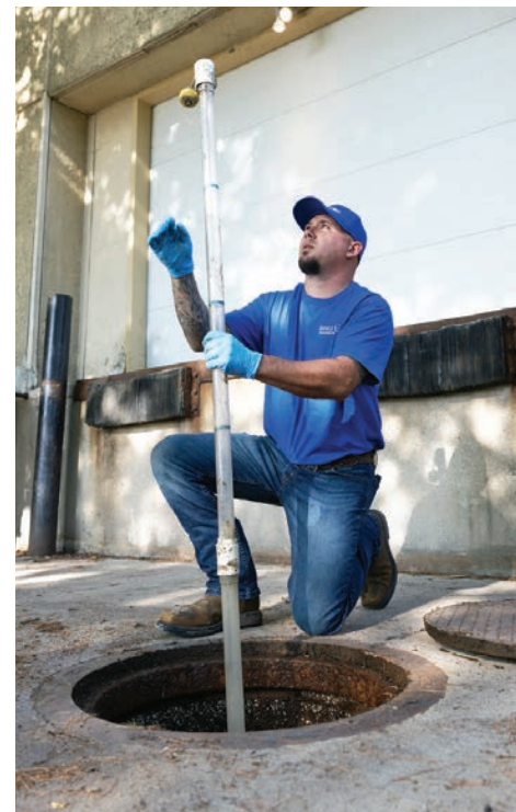
» Behle team lead Adam McDowell measures settled solids in a grease trap.
