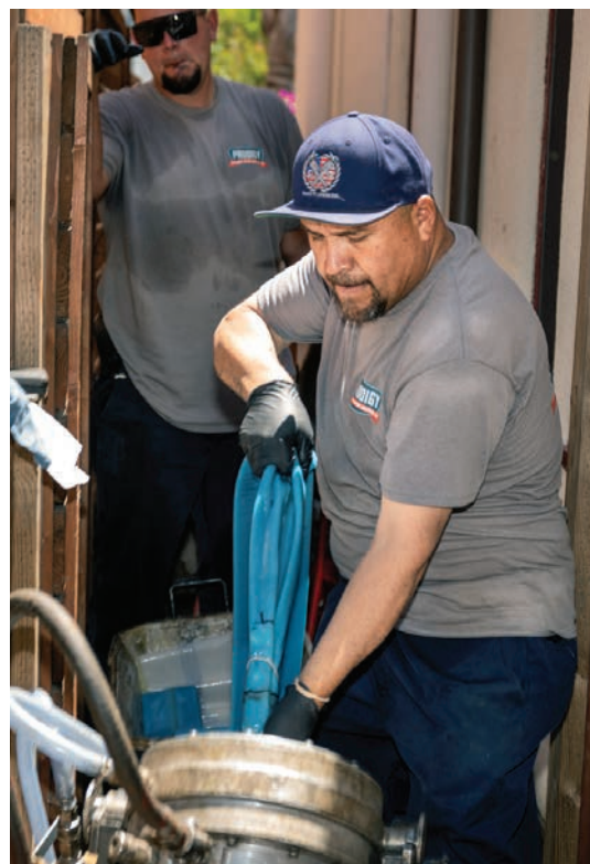
« Flores inserts a liner into an inversion machine.
