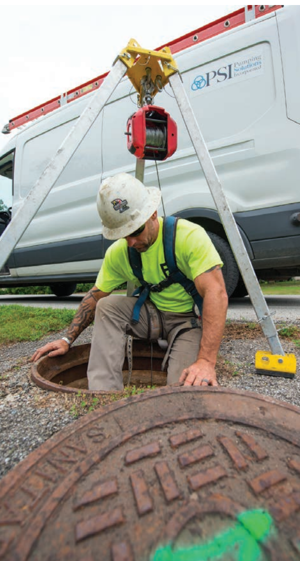
▲ Dustin Bailey enters a manhole to inspect a sewer line.
