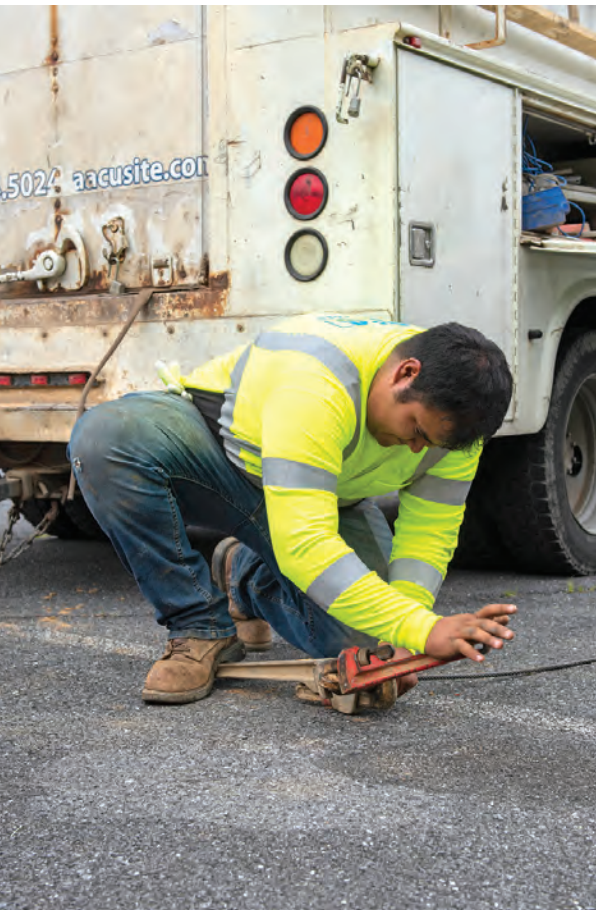
Ever connects hoses on a job site.
