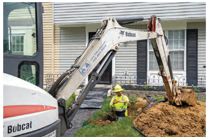
➤ Raul finishes digging the access pit for a pipe bursting job.
