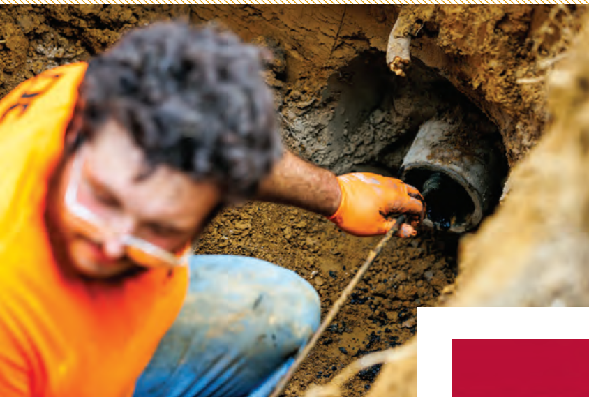
«Damian Pringle inspects a sewer line on a pipe replacement job.
