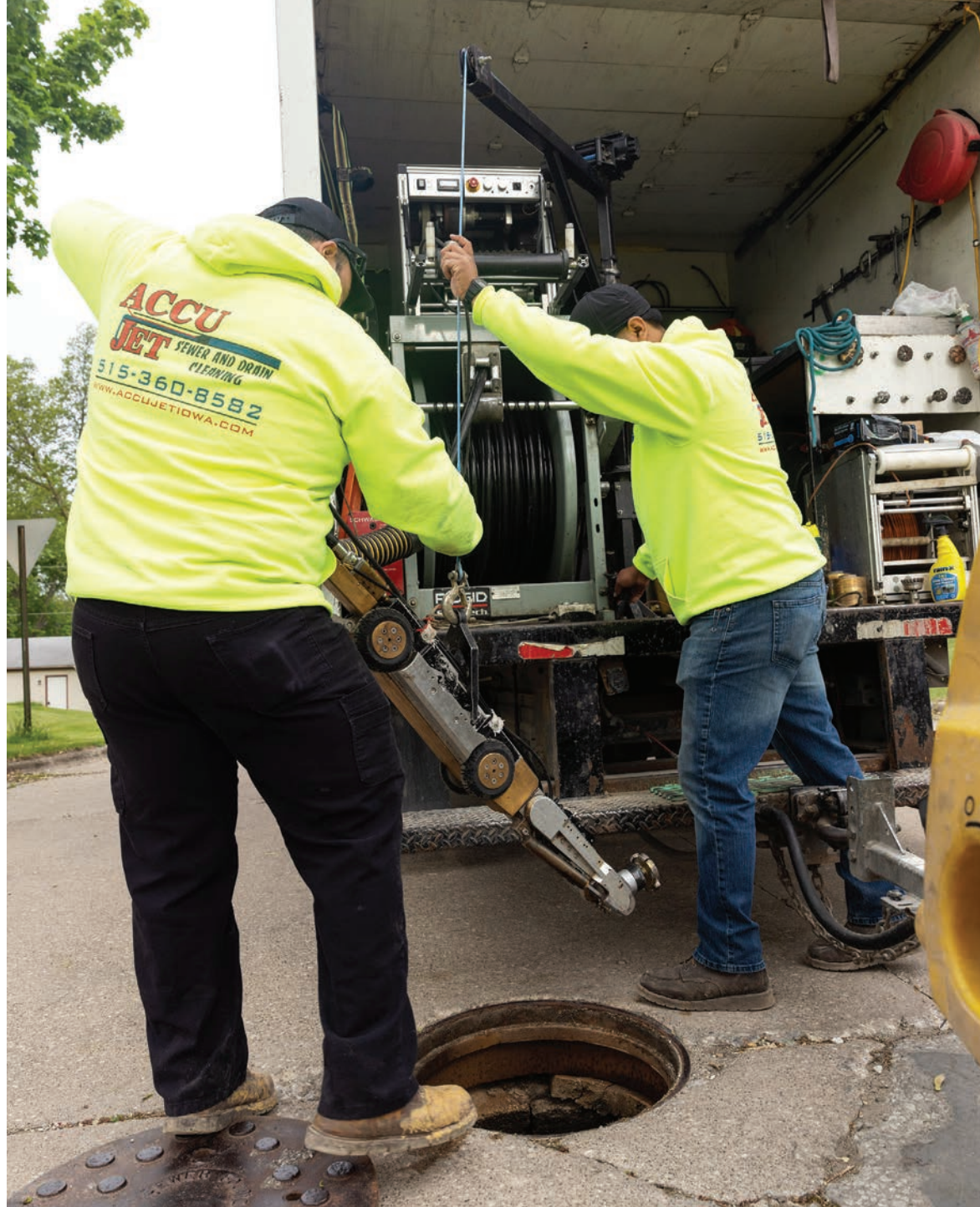
Technicians Jimmy Light, Eddie Cortes and Matt Elliott (from left) remove a manhole cover to inspect a sewer line.
