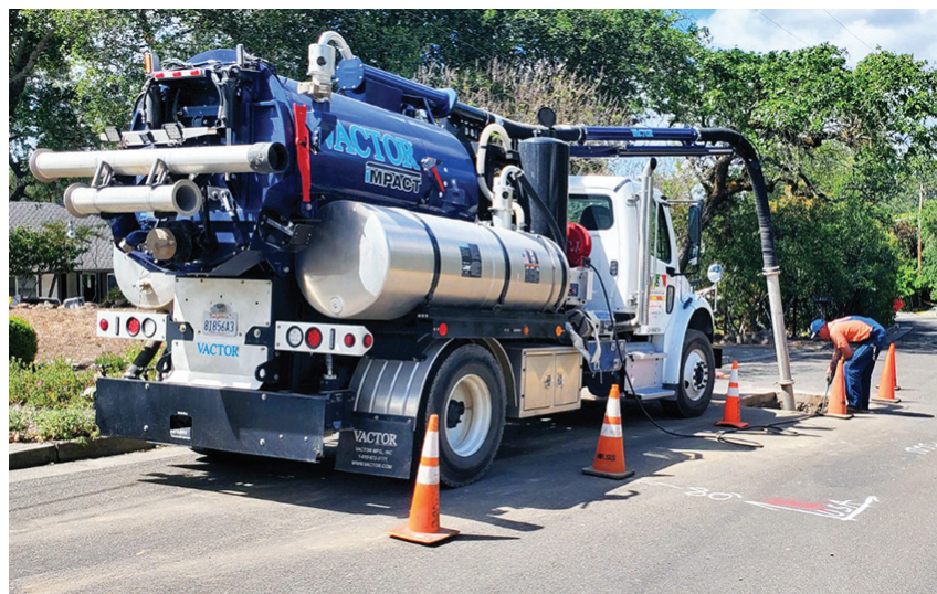
▲ Miksis Services operator Ivan Iverson uses hydroexcavation equipment on an iMPACT combination sewer truck built by Vactor to expose a sewer main in Healdsburg, California.
