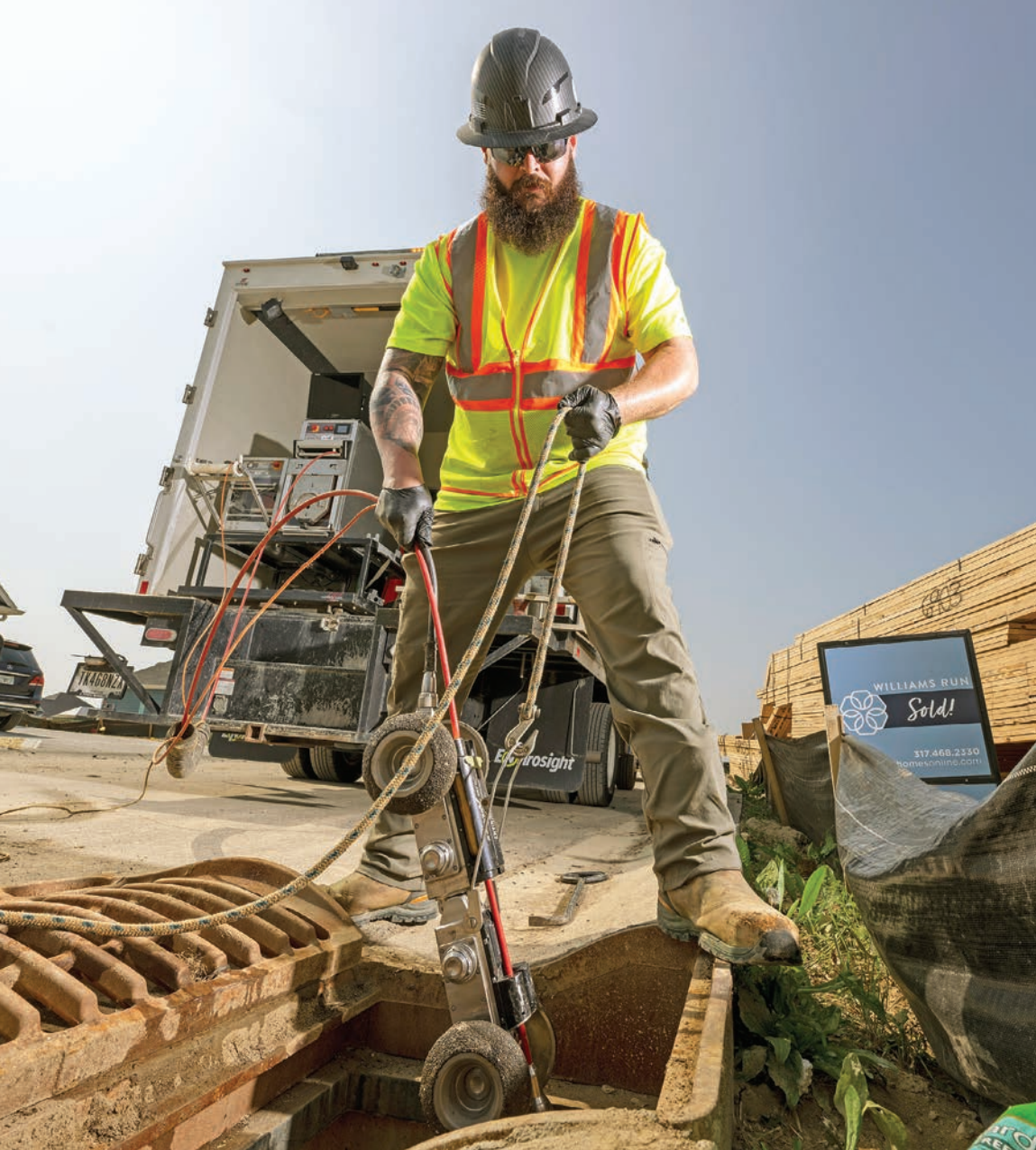
« Project manager Zach Fink lowers an EnviroSight SAT II lateral launch system into a storm drain.
