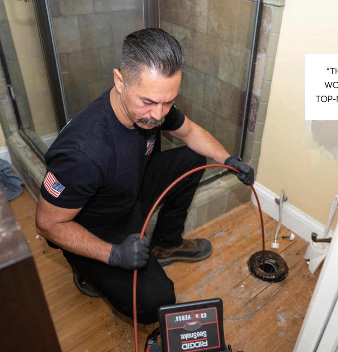
▲ Mike Lomonaco uses a RIDGID SeeSnake CS6X to inspect a toilet drain at a residence in San Clemente, California.
