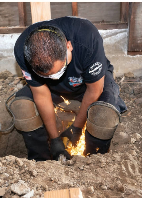
Lead lineman Orlando Alvarado prepares a pipe for a new fitting.
