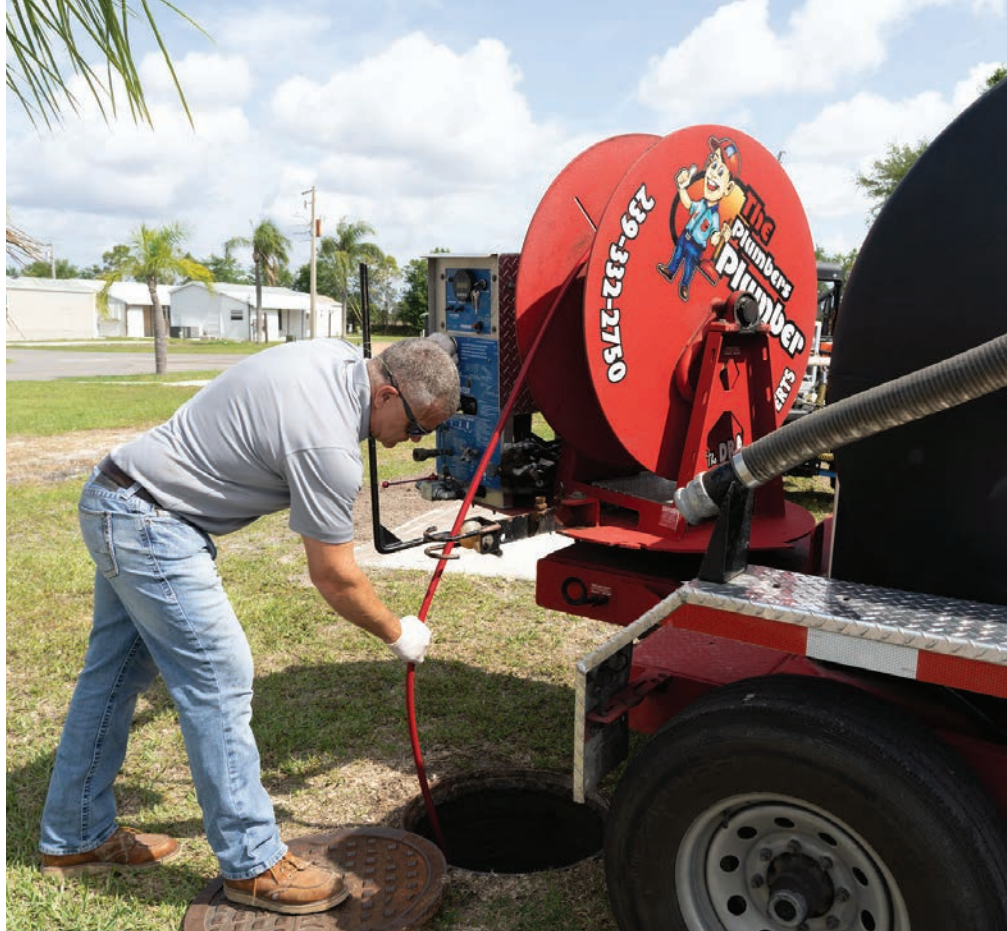
▲ Hedge feeds hose from a PipeHunter jetter into a sewer line.
