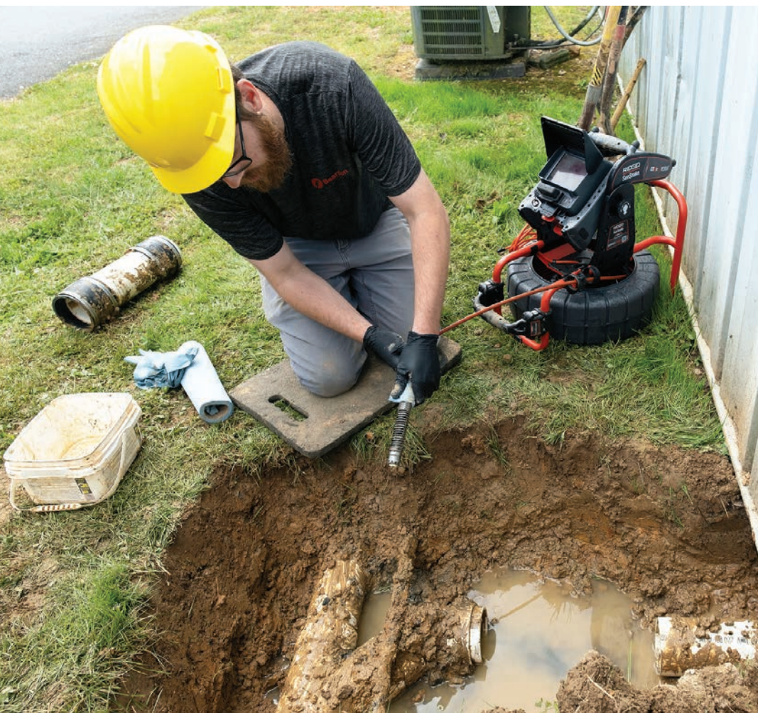
▲ Cody Letner wipes down the camera head of a RIDGID SeeSnake Compact C40 inspection system as he removes it from a pipe.
