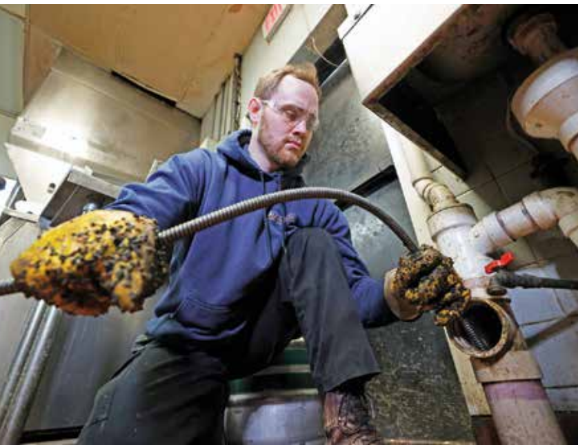
« O'Keefe snakes a drainline at a commercial job site.
