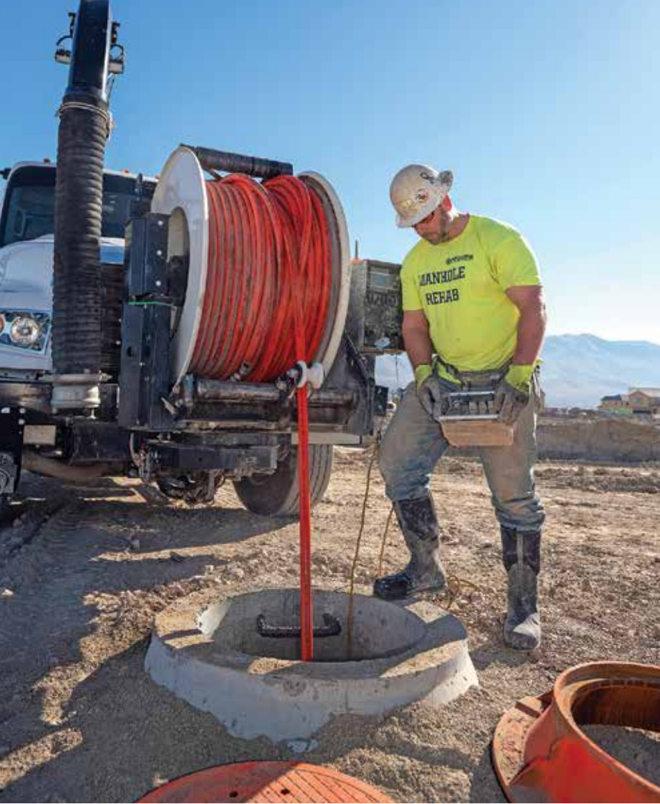
Technician Adam Stevenson jets a sewer line before a camera inspection.
