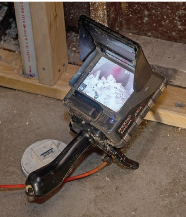
⚡ The descaling progress is shown on a RIDGID CS6x monitor.
