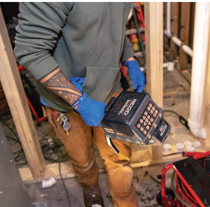
🔧 Delgadillo sets up a SeeSnake controller to inspect a drainline.
