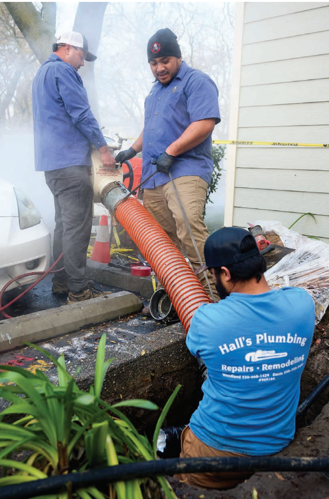
▲ The Hall's Plumbing lining crew prepares to shoot a liner into a residential lateral line.
