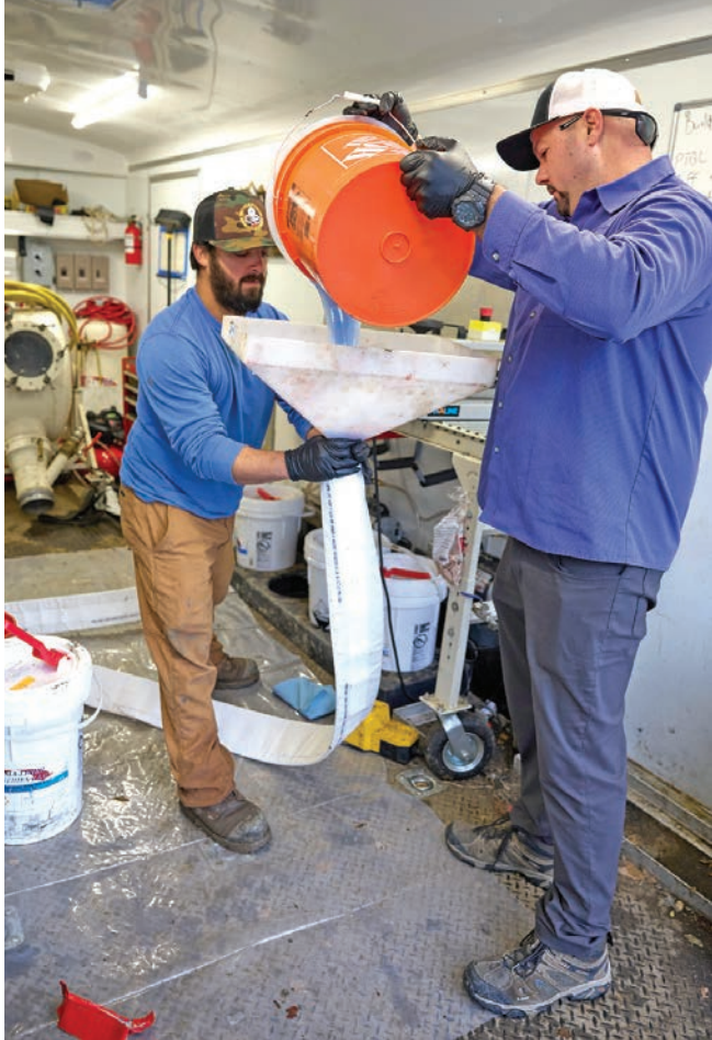
➤ Montoya holds the liner while foreman Joe Garin pours in the epoxy.
