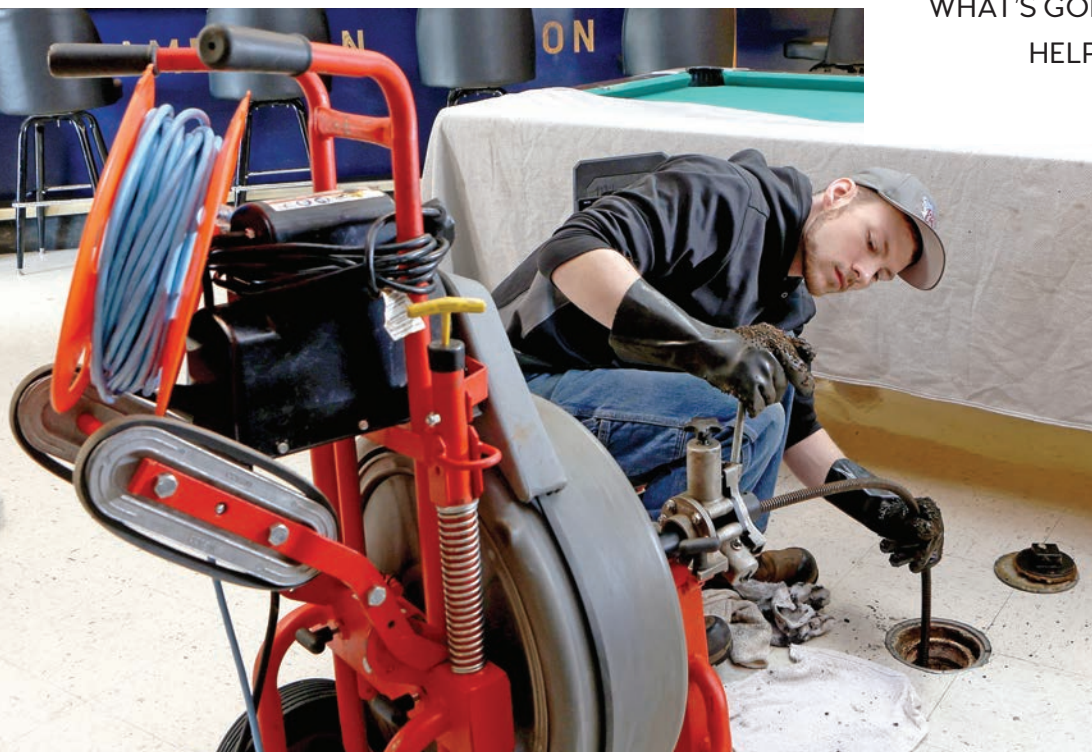
▲ Bowles feeds cable into a drainline to clear an obstruction.
