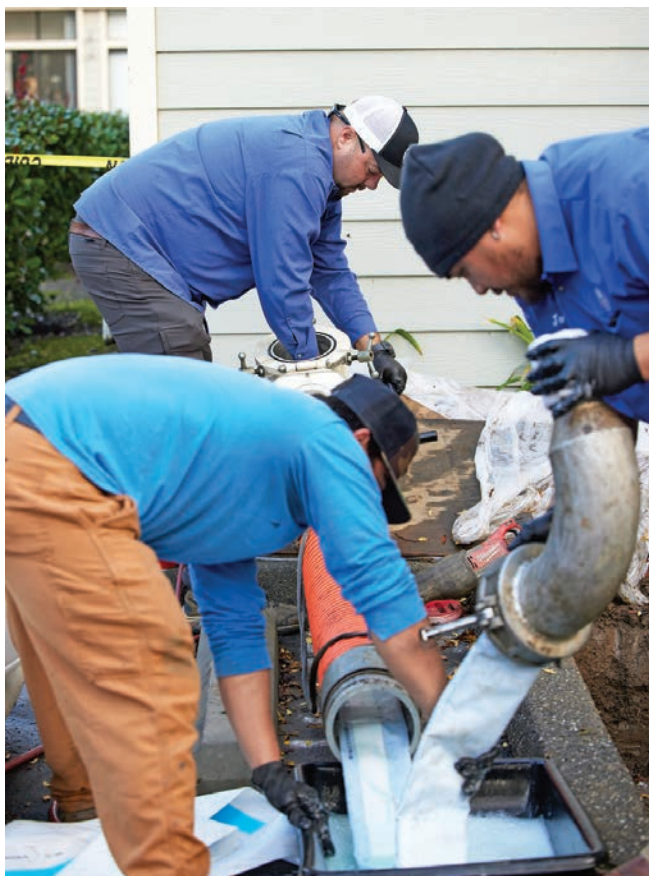
➤ Garin, Montoya and Kim position the liner and prepare to invert it into the line.
