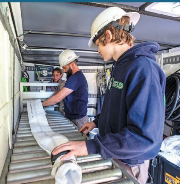
▲ Sonya Vasile, Jaco Vasile and Henryk Sucheck use a roller to make sure the epoxy mix is thoroughly pressed into the liner.
