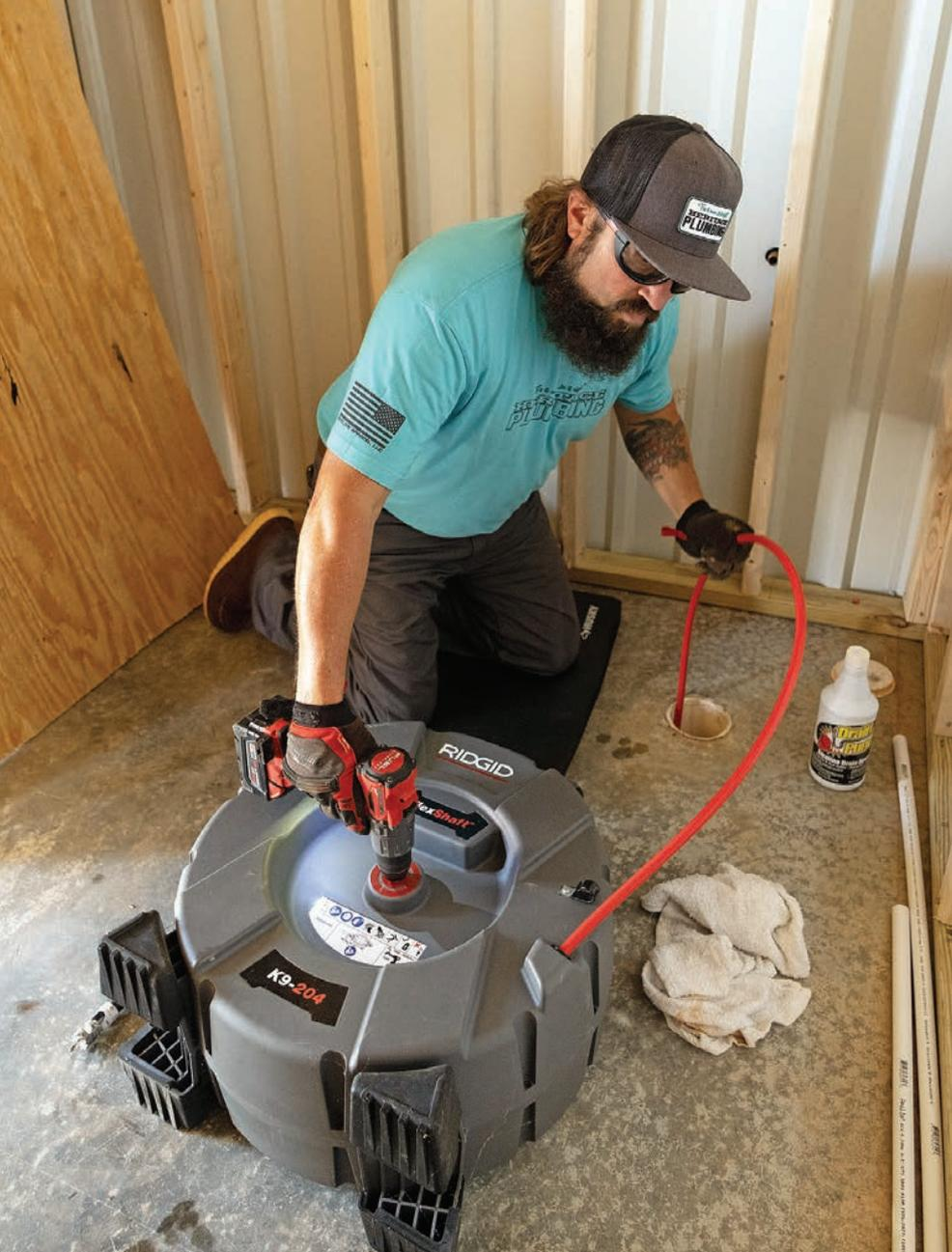
◀ Phillips uses a RIDGID Flexshaft K9-20 to remove debris and concrete from a sewer drainline.
