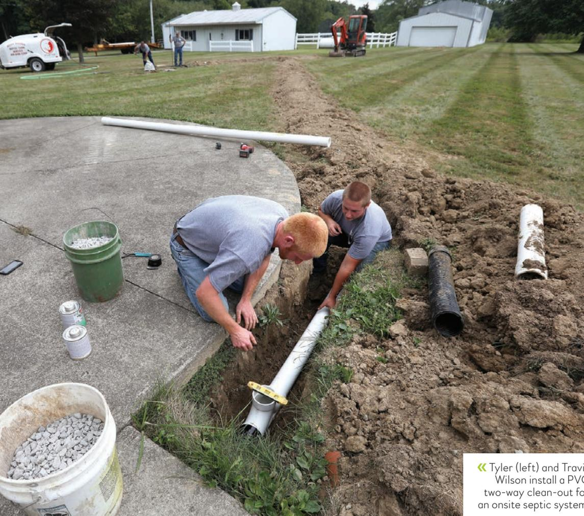
« Tyler (left) and Travis Wilson install a PVC two-way clean-out for an onsite septic system.
