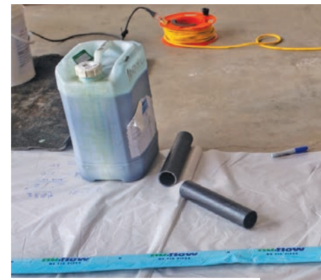
⤴ Rivera trims the NuFlow liner to the proper length.
