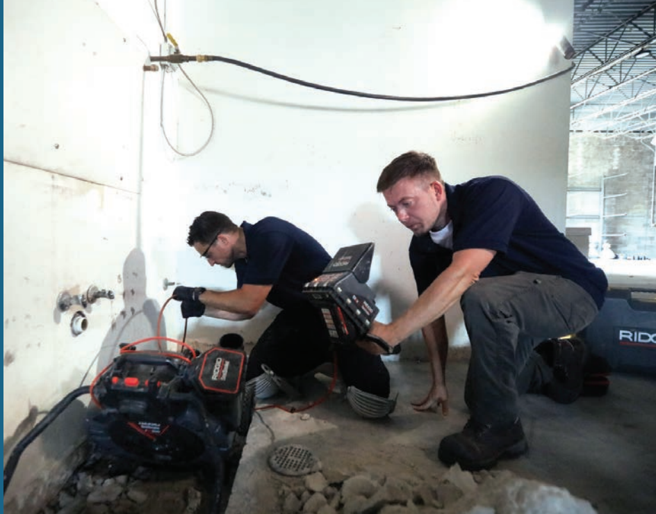
Chris Sbrocco (left) feeds the line as Belon watches the monitor while inspecting drainlines in a commercial building.
