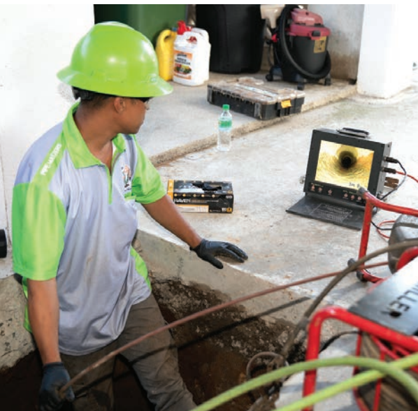
Devin Watabu checks a monitor as he inspects the line.
