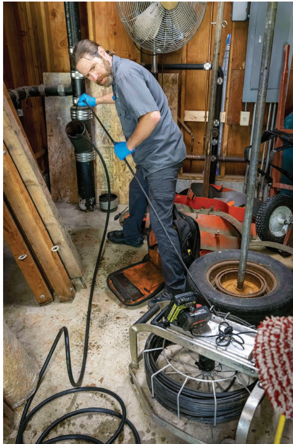
✔ Matthew Sadler works to clear a sewer lateral with a Warthog jetter nozzle, watching the progress with a Mini VU inspection camera from Insight Vision.
