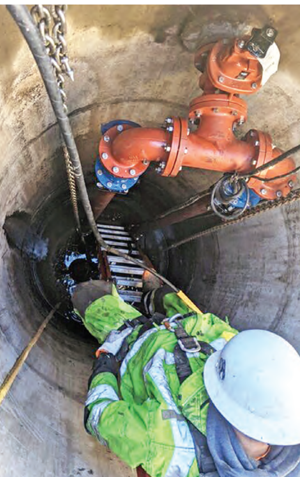
➤ A technician inspects the walls of a lift station prior to applying a lining.
