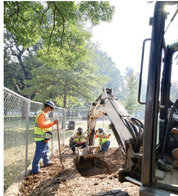
✔ Kirino Pacheco Luna, Anthony Ibarra and David Mendez (from left) guide Jose Pacheco Luna while excavating an access pit.
