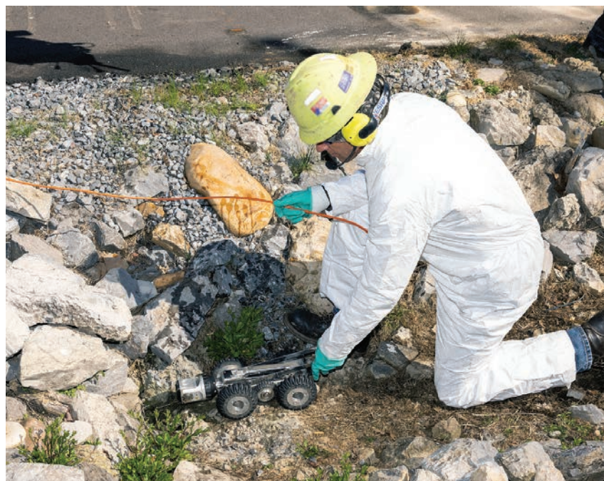
Andrew Davis uses a Sonetics headset to communicate with his crew member while preparing to send a Proteus crawler camera into a line to inspect it after cleaning.
