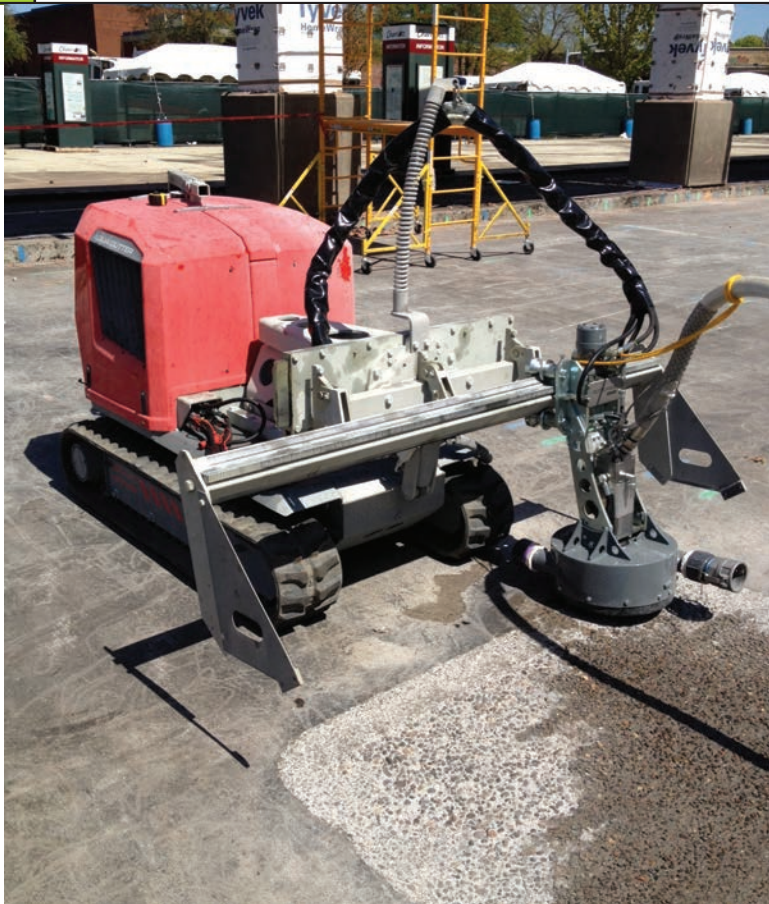
▲ For removing concrete, paint or other coatings, powerful hydrodemolition equipment provides maximum productivity compared to hand lances, due to the robot's ability to handle the higher water flow rates and reaction forces.
