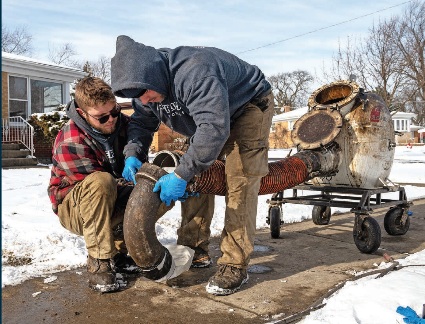
» Ron Richardson and Devin Snyder attach a loaded cal tube bladder to a Perma-Liner inversion drum.
