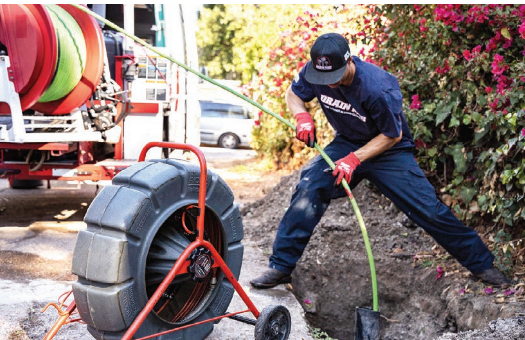
Joey Flores fires up a US Jetting 4018 trailer jetter to clean out a drainline on a residential job site.
