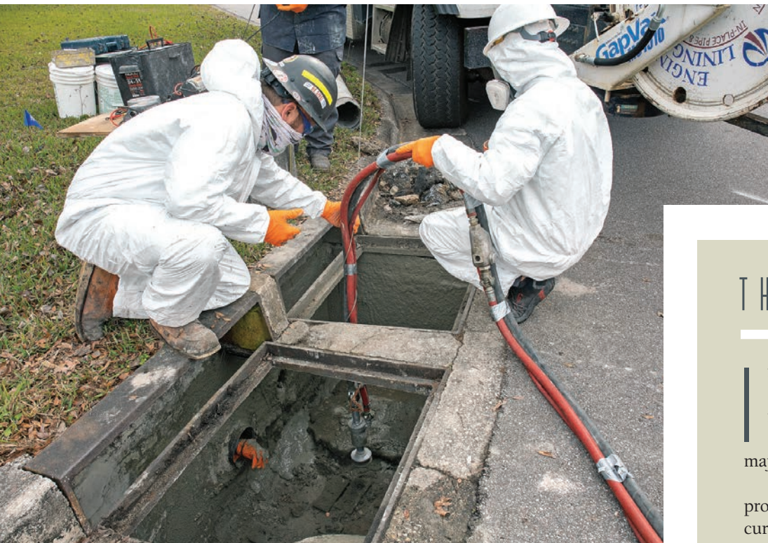
◀ Buddy Blake and Kyle Strickland begin a centrifugal cast application for a catch basin rehab project at the Orange Park Country Club.
