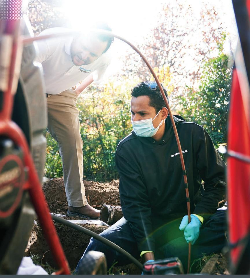
Trenchless Company crew leader Douglas Lagos uses a RIDGID camera system to monitor the progress of a Picote Maxi Miller prepping a residential sewer pipe for relining, while owner Max Greenberg looks on.
