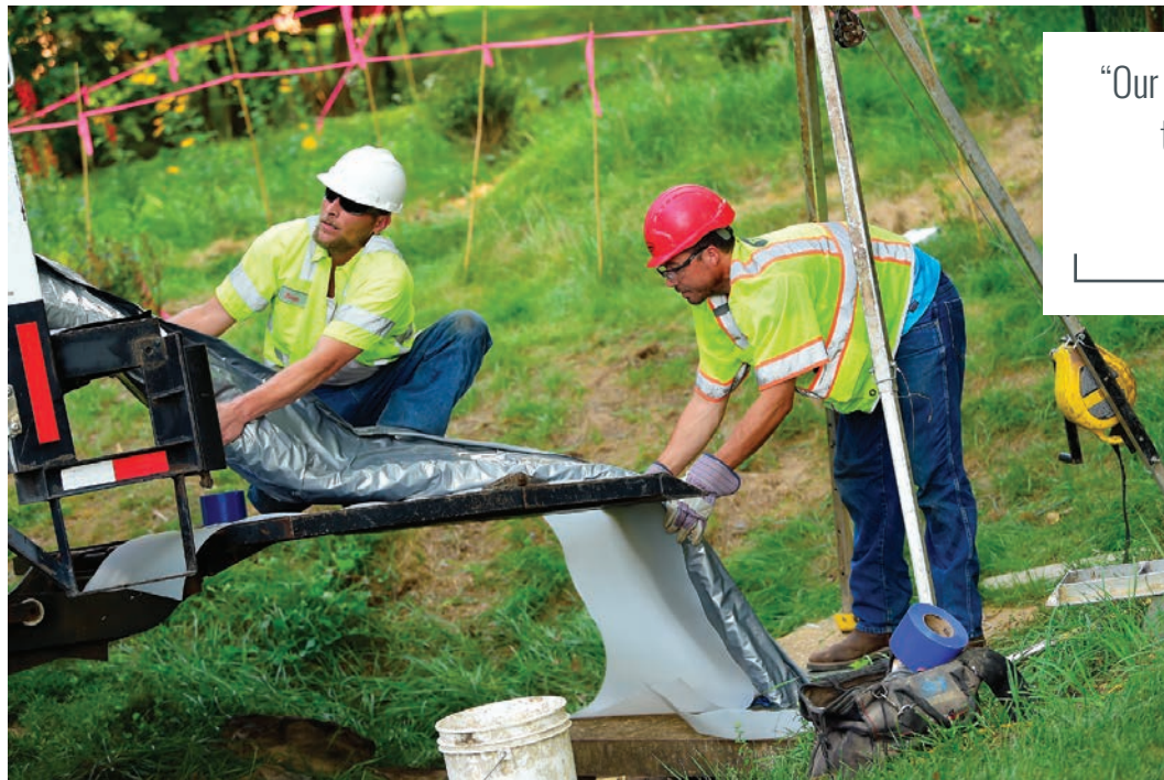
▲ Jeremy Houser (left) and Julio Ramos feed a new 18-inch-diameter, 311-foot non-styrene UV-cured Alphaliner into a stormwater line in McLean, Virginia.
