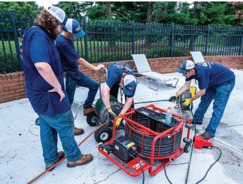
➤ Austin, Mike, Vinny and Ray (from left) use a jetter with a Warthog nozzle, a Maxi Miller with a diamond grinding head, and a Vivax camera simultaneously as they clear roots and debris from a pool deck drainline.
