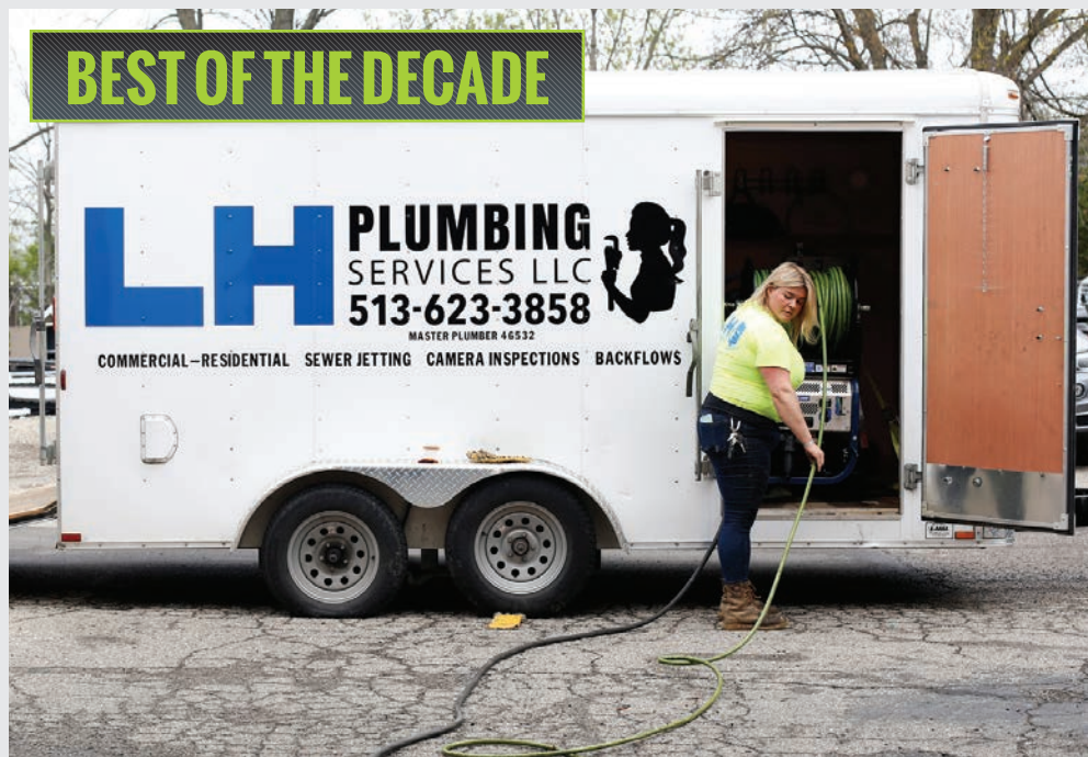
▲ Linda Hudek, owner and operator of LH Plumbing unspools hose from her jetter (Jetters Northwest) to clean a sewer line at a commercial property.
