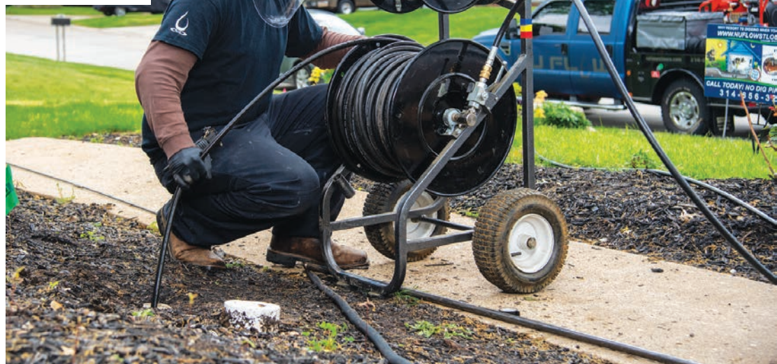
Technician Eric Turner cleans out a lateral line with a Spartan Tool jetter.
