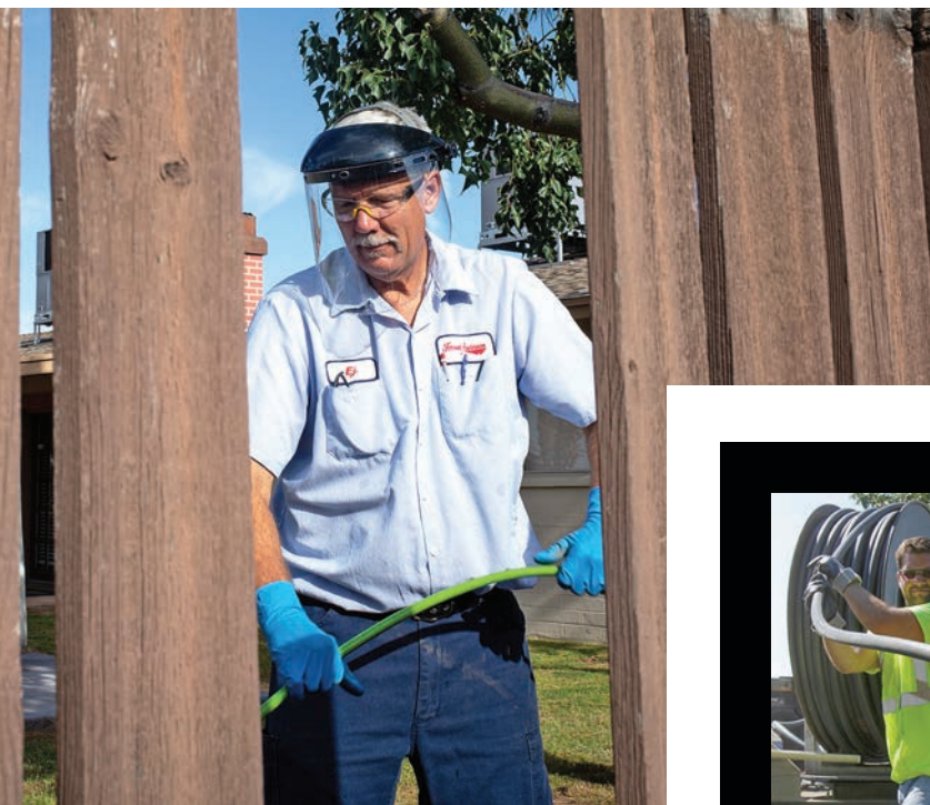
« E.J. Knowls feeds a jetter hose into the backyard clean-out of a residential lateral line.
