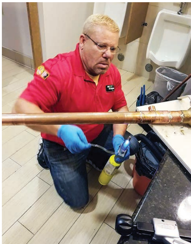
« George Garner solders a fitting for a bathroom remodel job.
