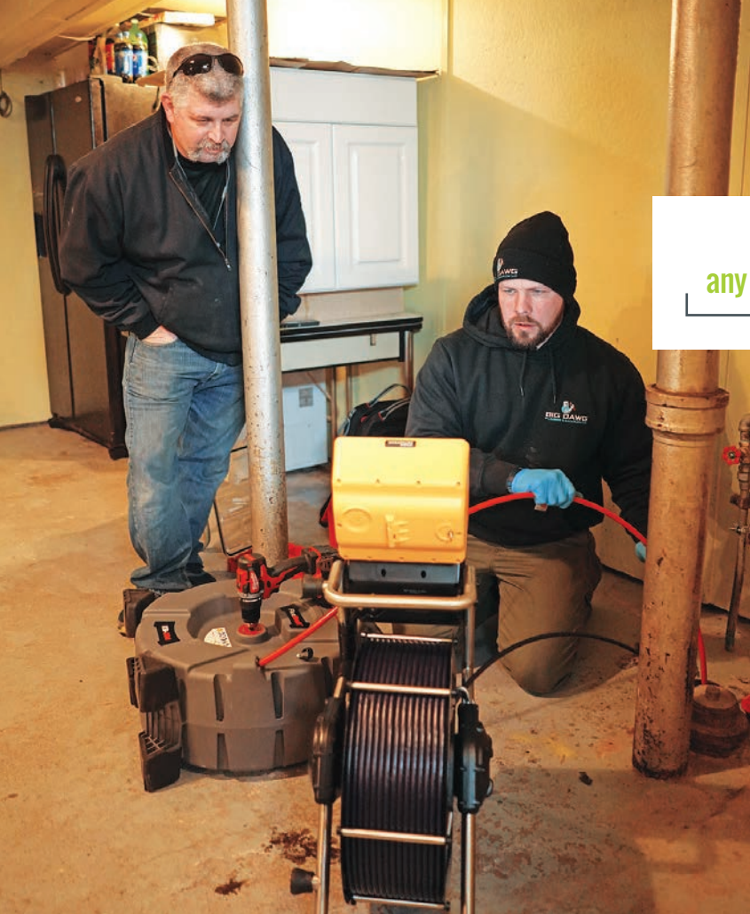
Michael Reed (right) and homeowner Butch D'Agostino watch the camera monitor while Reed cleans and inspects D'Agostino's basement sewer drain.
