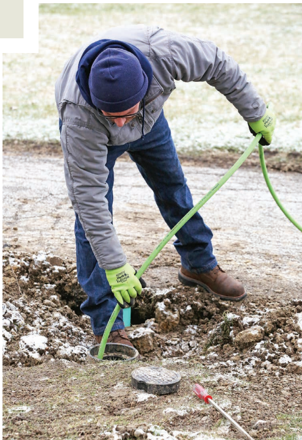
Technician O'Brien sets up a 2015 Spartan Warrior jetter (above) to clean a later line (below) at a home in Eastlake, Ohio.
