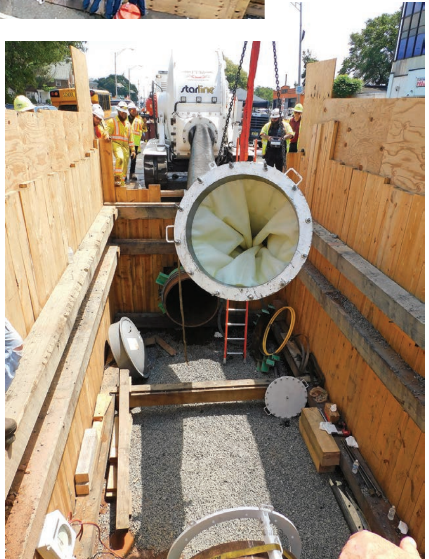
➤ The liner is moved into place to rehabilitate the cast iron gas main along Central Avenue in East Orange.
