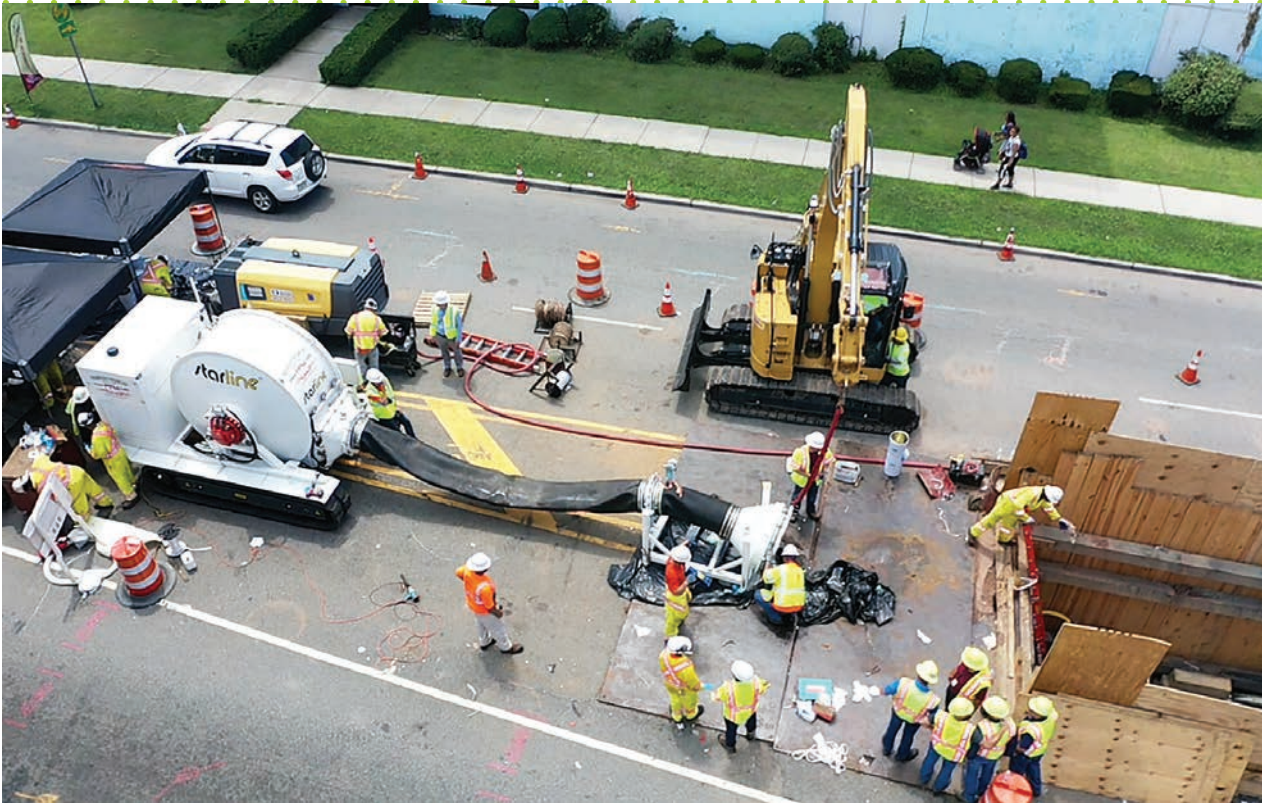
👁️ A bird's-eye view of the PPM crew, starline system and pit during the lining of a 42-inch natural gas main in East Orange, New Jersey.
