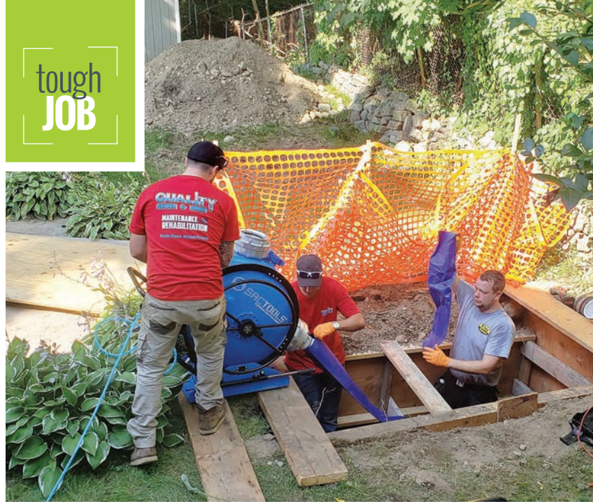
Brian Dacey, Russell Joe and Johan Lindholm prepare to shoot a liner through a calibration tube that keeps it from expanding.
