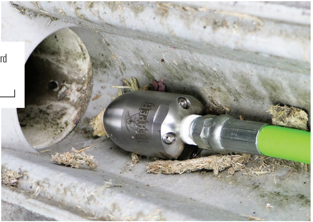
Hydra-Flex offers five different Reaper models; Midland owns a 9 gpm model with a 3/8-inch inlet connection, designed for 3- to 6-inch-diameter lines. The rotating front jet creates a 24-degree cone of coverage.
