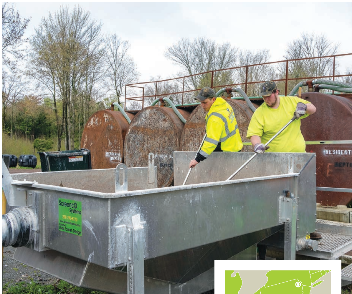
Sean Durango and Josh Hartman remove debris from a Maxi Screen 400 receiving station (ScreencO Systems) while a vacuum truck off-loads septage.
