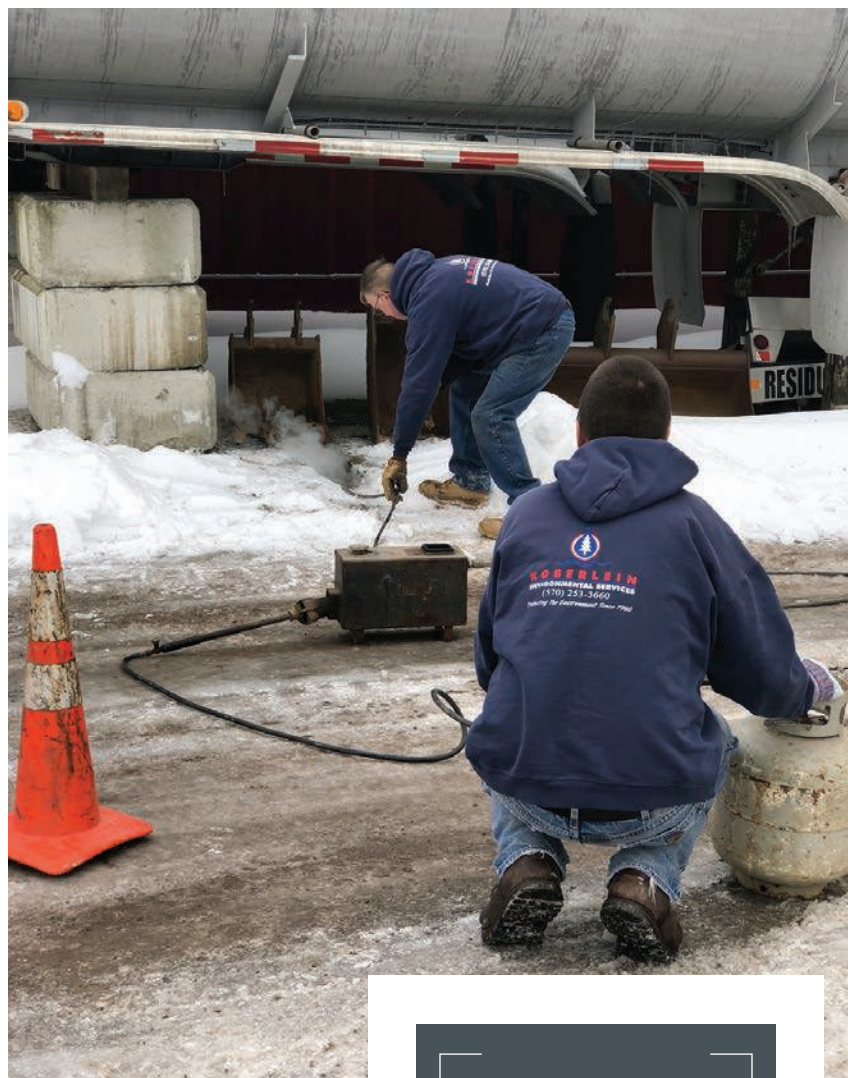
➤ Gary Sprague, general manager at Koberlein Environmental Services, and Gene Mohrmann, operations manager, use an Arctic Blaster to thaw out a 4-inch drainline at a business in Honesdale, Pennsylvania.
