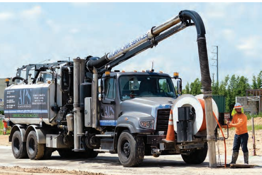
« David Reyes operates the Vacall truck while cleaning a sewer line.
