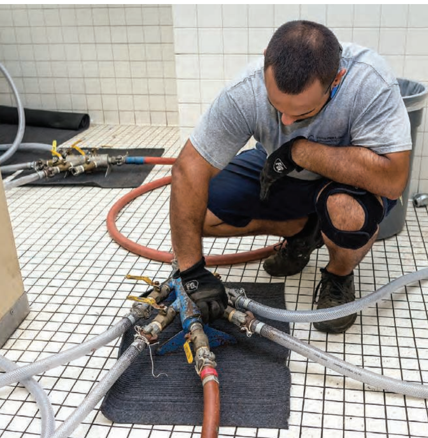
➤ Tristan Bourdier connects ePIPE fittings to an ACE DuraFlo manifold.
