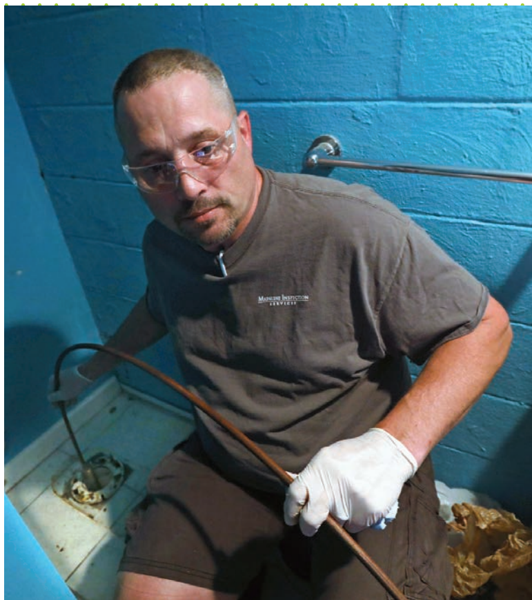
⚡ Hooper feeds the camera into the clogged line through a basement shower drain.
