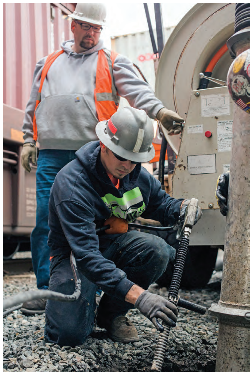
Hydroexcavation safety takes planning and teamwork. Having a second person on site to watch the operator and keep an eye on everything is critical. (Photography by David Ryder)
