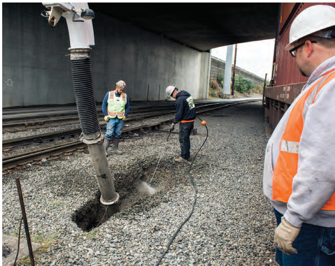
▲ One of the biggest concerns in hydroexcavation is boom clearance. While operators are focused on the ground before them, booms are stretching far overhead and can come in contact with power lines or other obstacles if not closely monitored.
