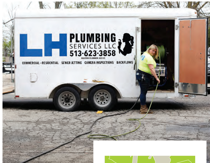
▲ Linda Hudek, owner and operator of LH Plumbing unspools hose from her jetter (Jetters Northwest) to clean a sewer line at a commercial property.
