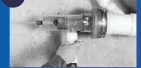
OPEN VALVE AND DRAIN CONTENTS
