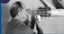
CLAMP TO CLEAN OUT DRAIN
