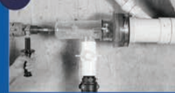
CUT HOLE IN DRAIN CAP
