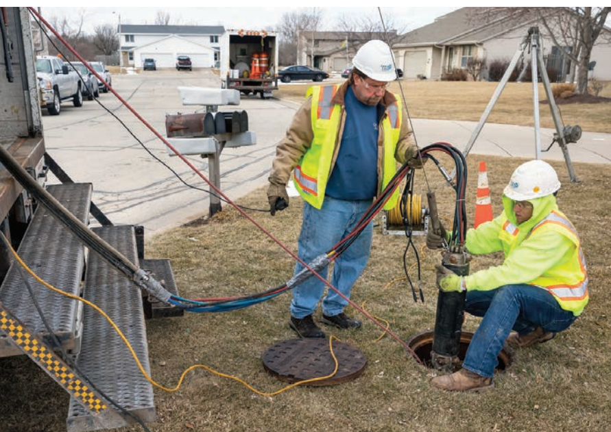
Greg Healy, co-owner of Wisconsin-based Great Lakes TV Seal, lends a hand to Hunter Strick (right) while grouting a lateral connection in a sewer main with an Aries grout truck.
