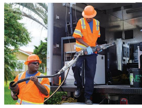
All inspection camera systems are sealed in some way to protect sensitive components from harsh environments. They can be protected from moisture and water through pressurization with an inert gas, or through design standards and are tight enough and strong enough that you don't need to worry about pressurizing the inside.
