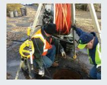
RESULT / "I had a big root clean-out problem, and I found out the Vacall delivered a higher level of performance to power the chain cutter down in the 24-inch mainline," Fox says. "The Vacall delivers 87 gpm at 2,000 psi, so it does a good job chopping up heavy root networks and washing them away." 330-339-2211; www.vacall.com. c
