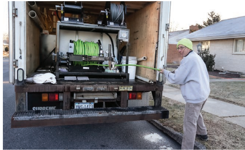
Mike Leonard pulls hose off his truck-mounted HotJet USA jetter to clean a clogged lateral line.
