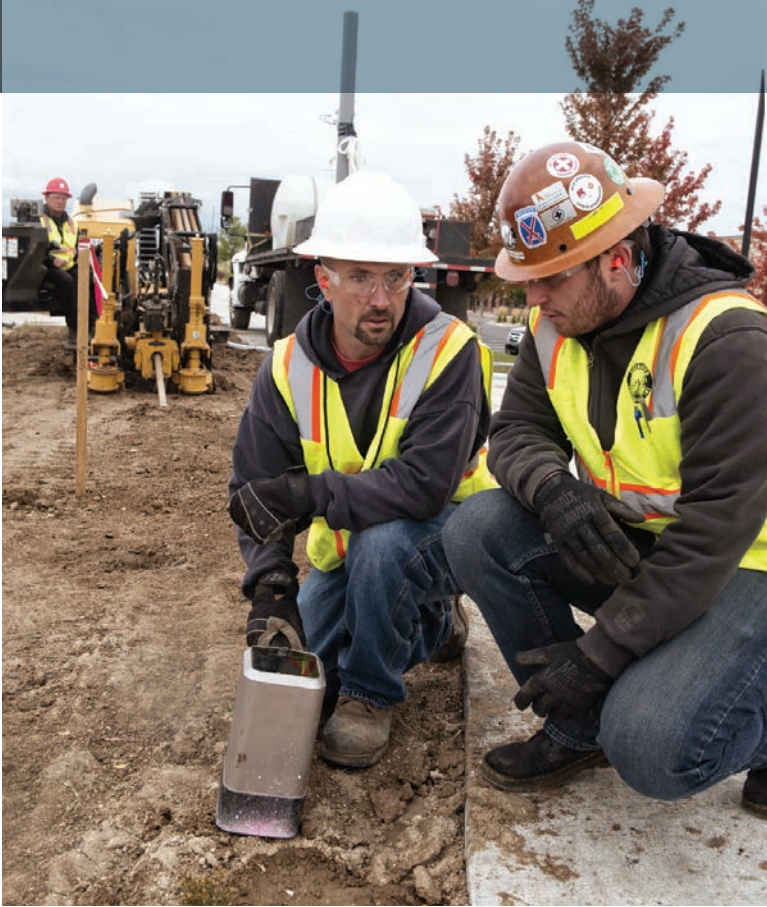
Supervisor Josh Allen (right) and head locator Branden Witt evaluate the signals from a Digital Trak F5 walkover locator to assist drilling operator Mike Canandy on a directional drilling job.
