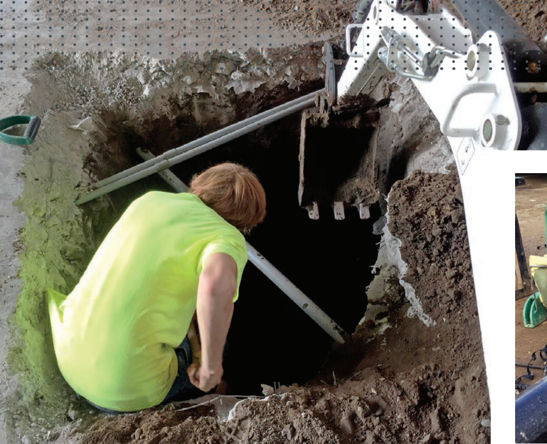
◀ A worker hand-digs around buried utilities on a lateral repair job.
