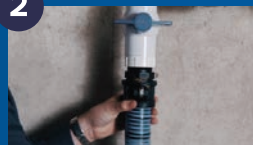
ATTACH DRAIN HOSE
