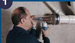
CLAMP TO CLEAN OUT DRAIN
