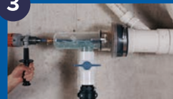
CUT HOLE IN DRAIN CAP
