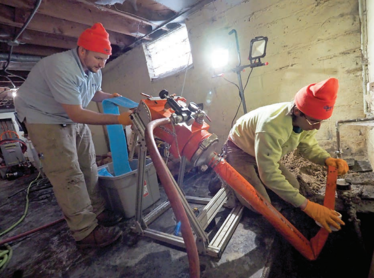
Ben Smith (left) feeds the end of a liner into the inversion unit while technician Alex Pannez gets set to guide it into a lateral cleanout.
